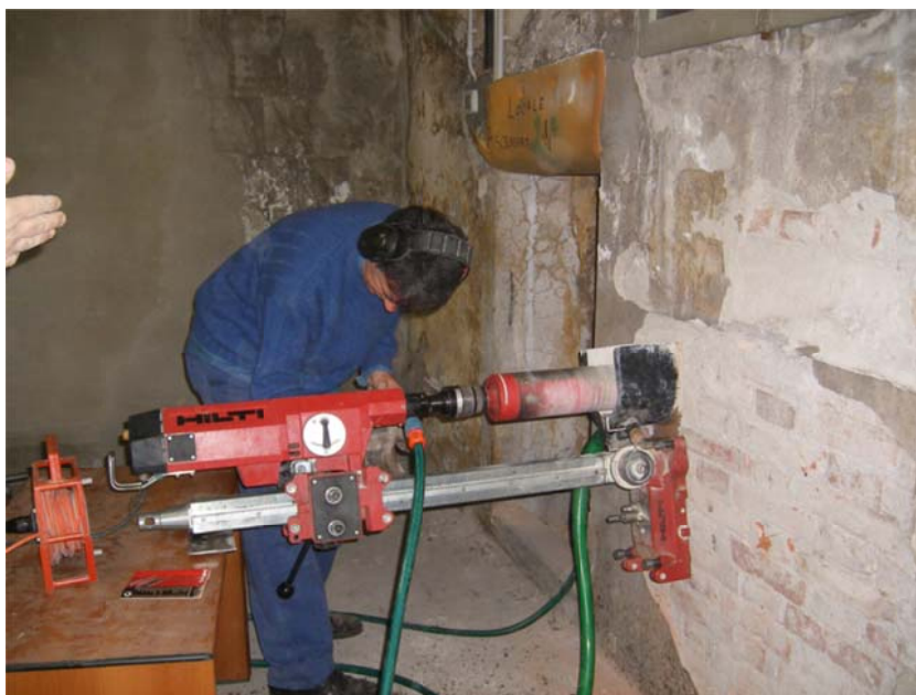
Figure 4.2 Core drilling during an in-situ experimental campaign
