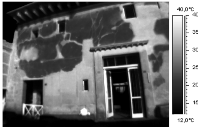
Figure 2.23 Thermography overview of a building façade (Colla et al. 2008).
