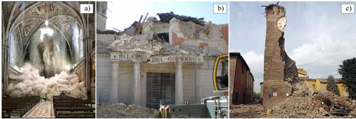
Figure 1.1 Effect of earthquake on masonry structures: Basilica of Saint Francis in Assisi, Italy in 1997 (a), Prefecture Palace in L'Aquila, Italy in 2009 (b) and Clock Tower in Finale Emilia, Italy in 2012 (c).
