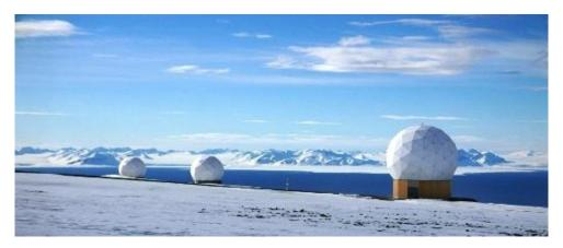
Figure 45. The Metop satellites are operated via two CDAs collocated in Svalbard, Norway and linked to the operational ground segment in Darmstadt via fibre-optic and satellite communications links
