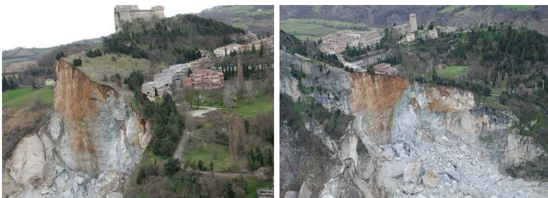
Figure 12. Views of the 2014 landslide, from the top views the closeness between the landslide crown and the buildings is evident
