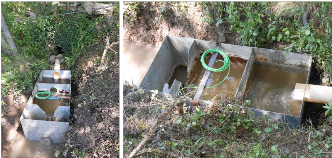
Figure 93. Discharge-gauge equipped with an electric transducer
