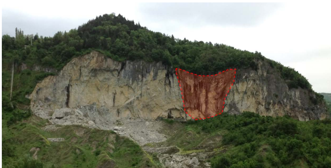
Figure 32. Highly fractured area in the Northern cliff. An higher degree of fracturing is indicated also by the presence of a higher amount of water circulation (highlighted by darker secondary deposits)
