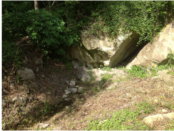
Figure 91. One of the main springs outflowing at the contact between the clay/shales and the rock slab
