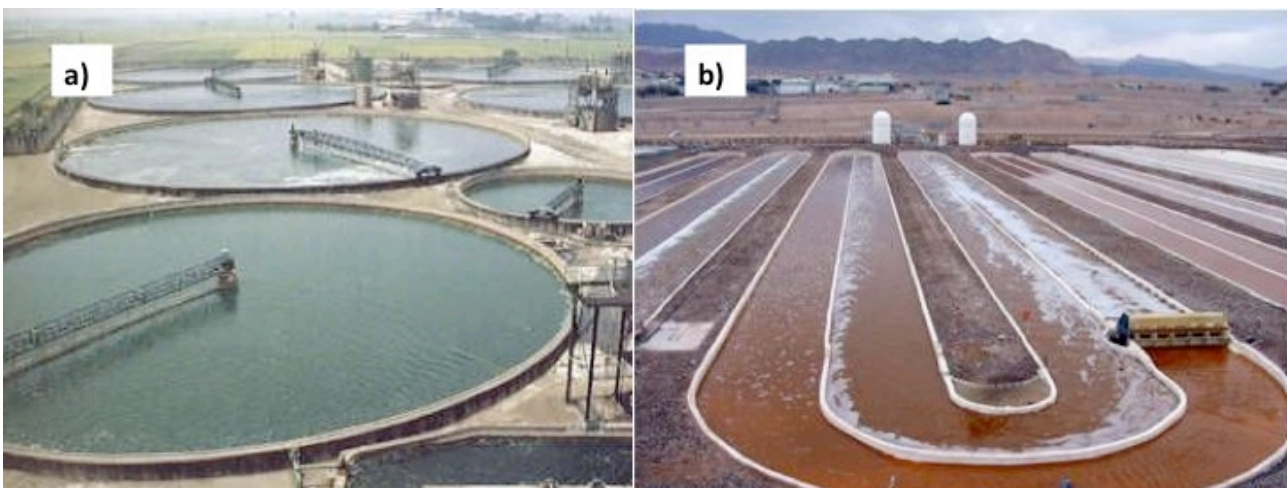
Figure 10 Example of open ponds: (a) Circular ponds in Asia; (b) Raceway ponds in Israel.
