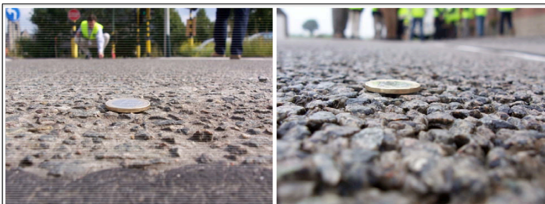
Figure 2.19 Exposed aggregate (left) and porous concrete (right) [62]
