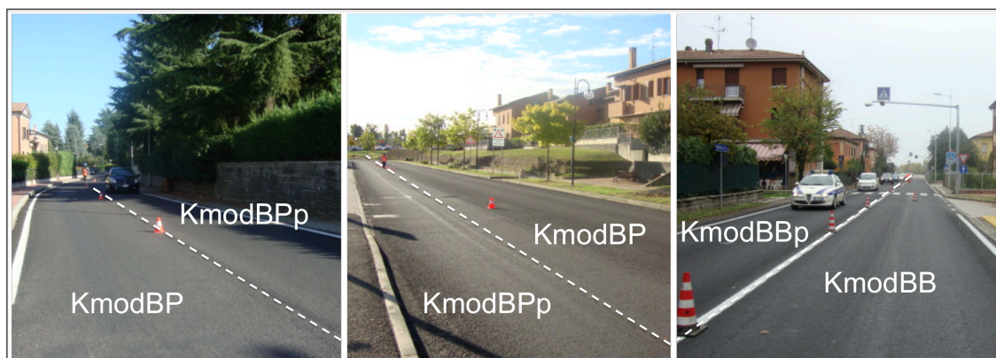
Figure 4.9 Multipurpose microsurfacing in Crespellano (left), Ozzano dell'Emilia (centre) and San Giorgio di Piano (right).
