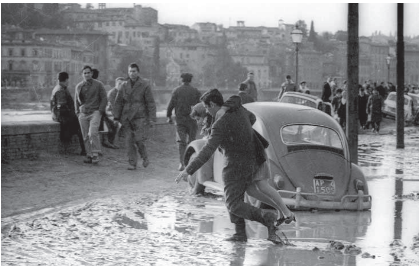
Note 2 The flood of '66 in Florence 2
