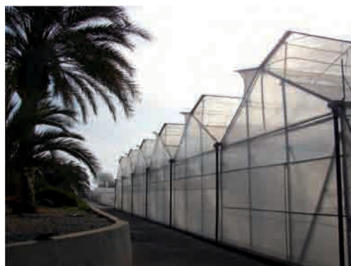
Plate 10 “Inversos” greenhouse. Prototype under evaluation. Fundacion Cajamar, Almería , Spain
