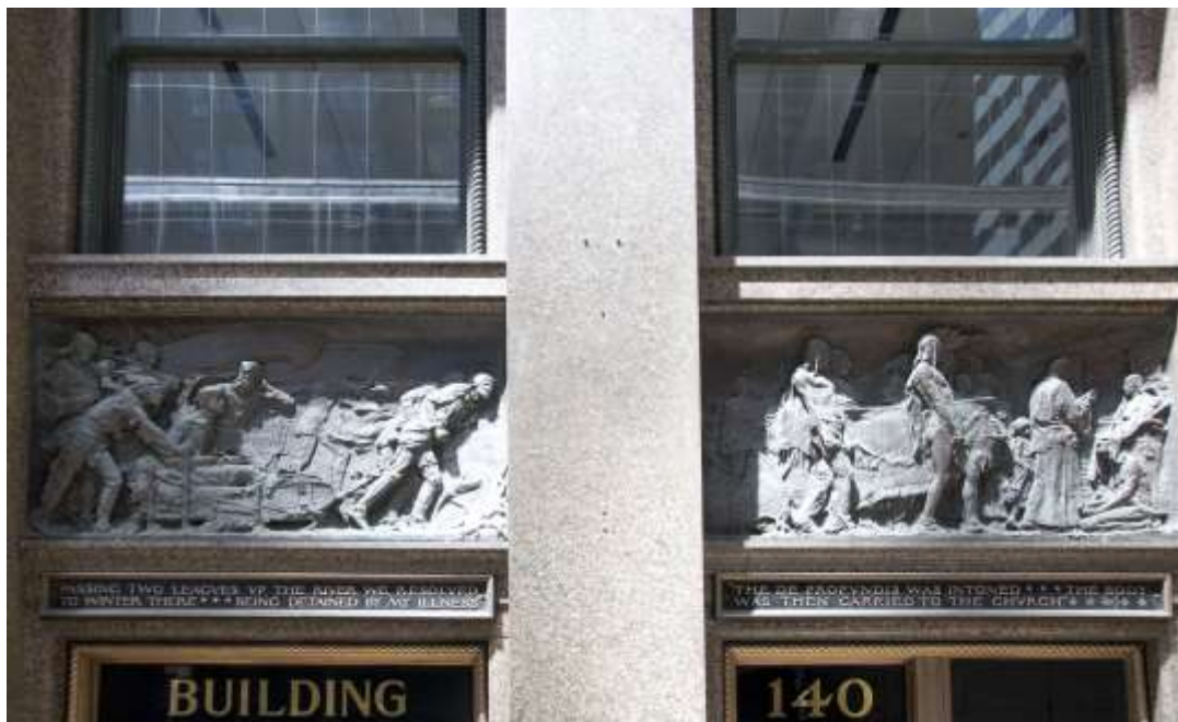
Figure 6.6 Holabird & Roche, Marquette Building, Chicago (1895); photo by author.
