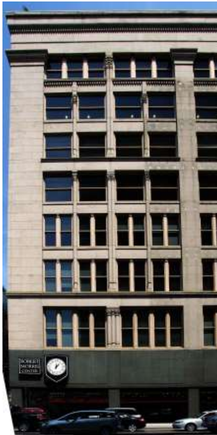
Figure 3.16 Jenney & Mundie, Levi Z. Leiter Building, Chicago (1891); photo by author.
