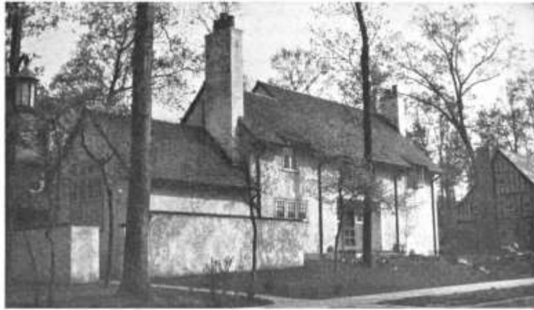
Figure 4.12 H. T. Lindeberg, Boardman Robinson House, from The Honest House (1914)
