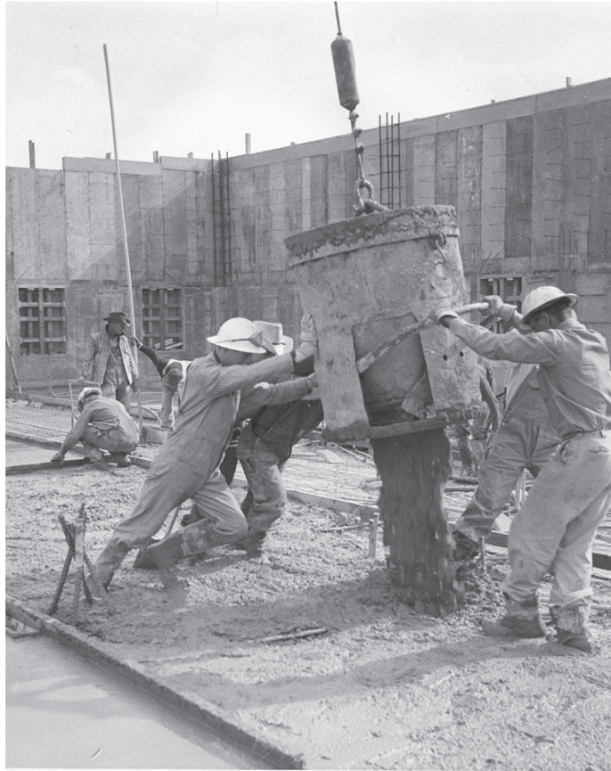
Figure 9: Construction workers pour concrete. Image Credit: Jackson Hole Historical Society
