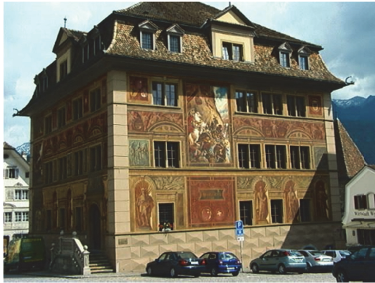
Figure 18: Schwyz Town Hall located in Schwyz Switzerland. “The murals are among the first examples of use of KEIM Mineral Silicate paints and have been retouched only twice since.”(Townhall and Murals in Schwyz, Switzerland). Image Credit: www.keim-usa.com
