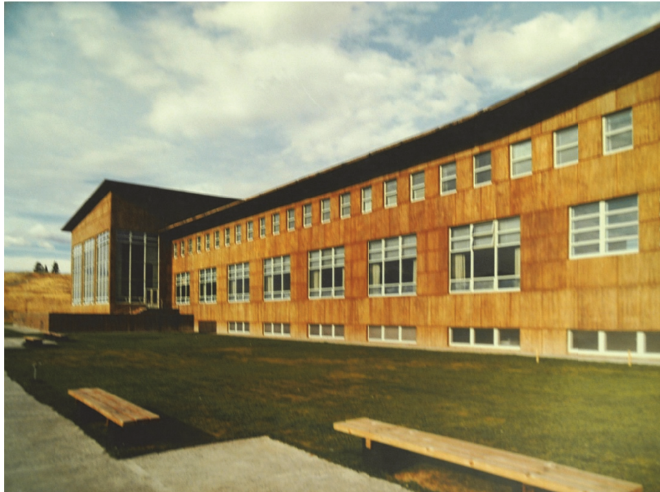
Figure 14: Appearance of the west elevation of the Central Building ca. 1960. Notice the red-brown hue of the stain and the variegation that allows the concrete to show through. Image Credit: Rockefeller Archives Center
