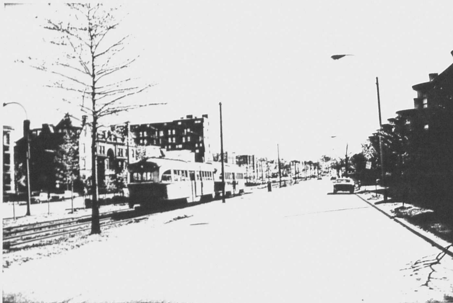
Figure 45. Wide Raised Median Along Beacon Street, Cleveland Circle Line
