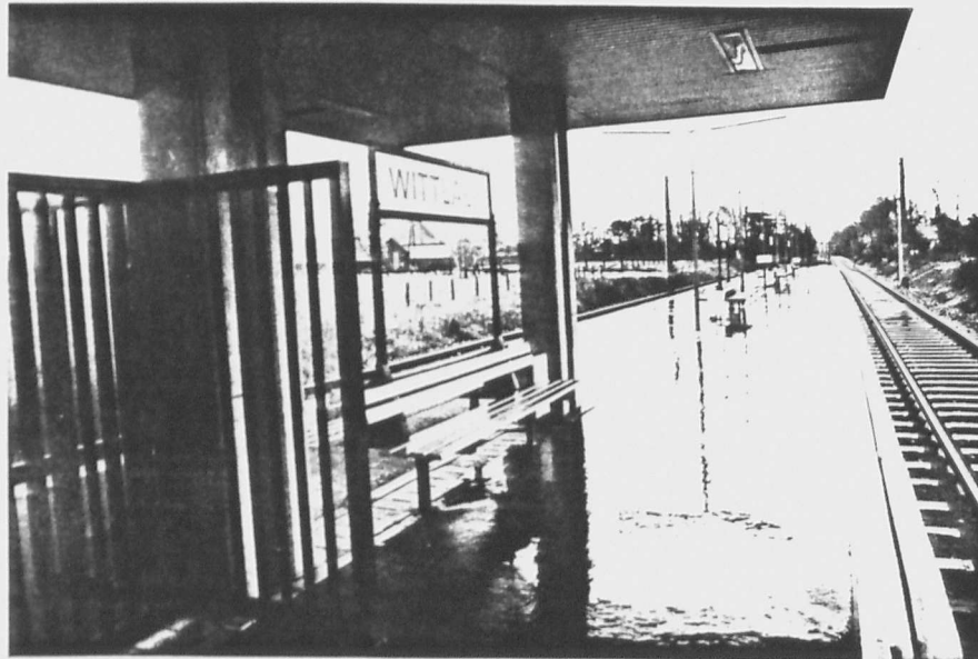
Figure 16. Wittlaer Station, Dusseldorf
