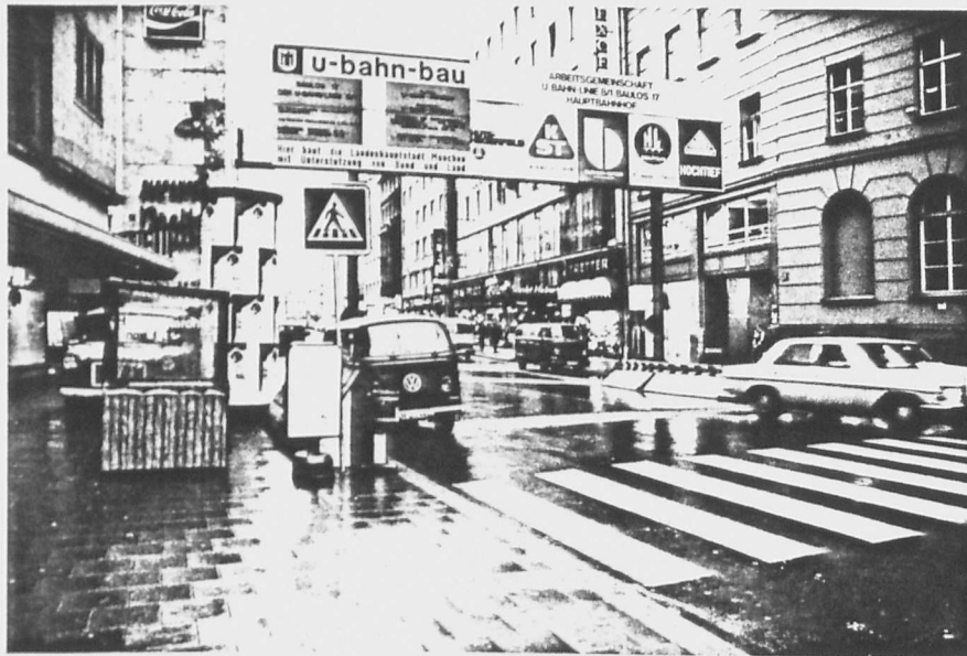
Figure 20. Sign at U-Bahn Construction Site
