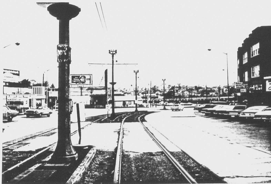
Figure 54. Contrasting Pavement on Media/Sharon Hill Lines, Red Arrow Division
