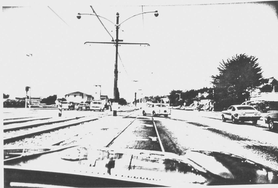
Figure 31. Double Left Turn Lane for Autos and LRT at 19th Avenue and Winston Drive
