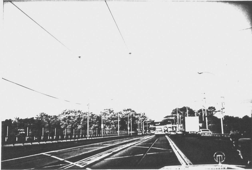
Figure 53. Painted LRT Median
