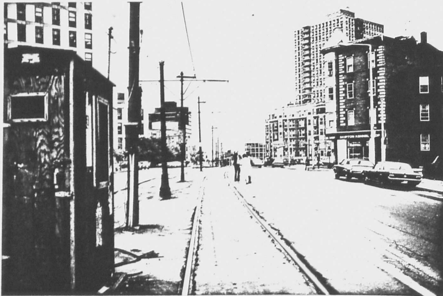
Figure 42. Narrow Median, Huntington Avenue, Green Line
