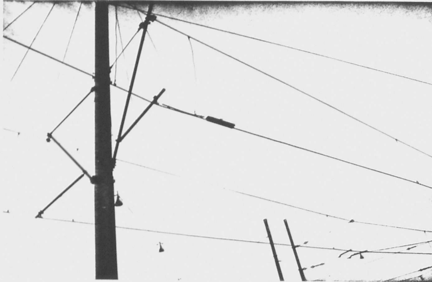
Figure 2. Overhead Detector used in Gothenburg
