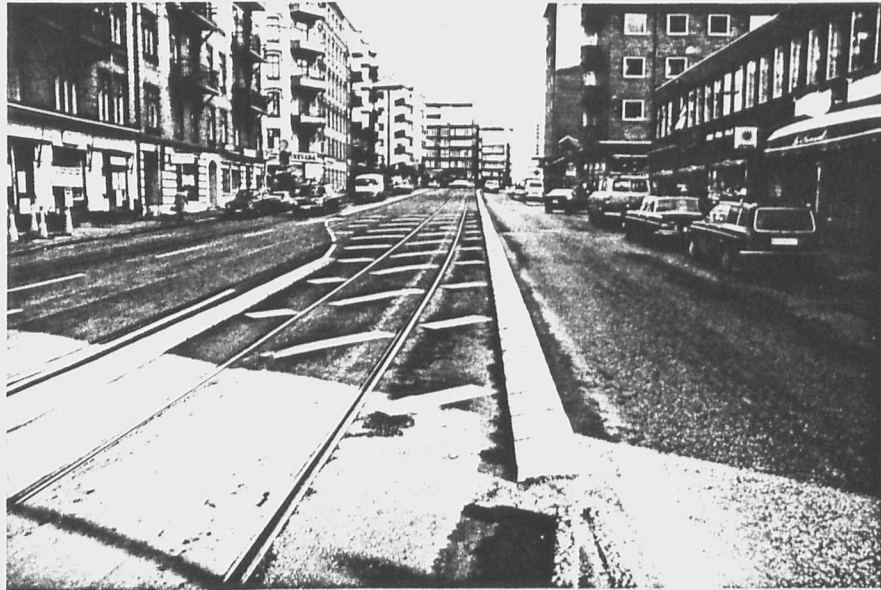
Figure 9. Line No. 3 Right-of-Way, Gothenburg
