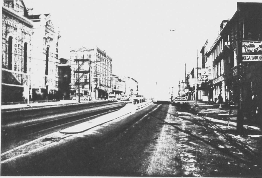
Figure 52. Raised Station Platform in Median
