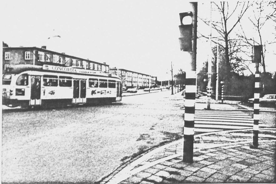
Figure 28. Line No. 9 Intersection, The Hague
