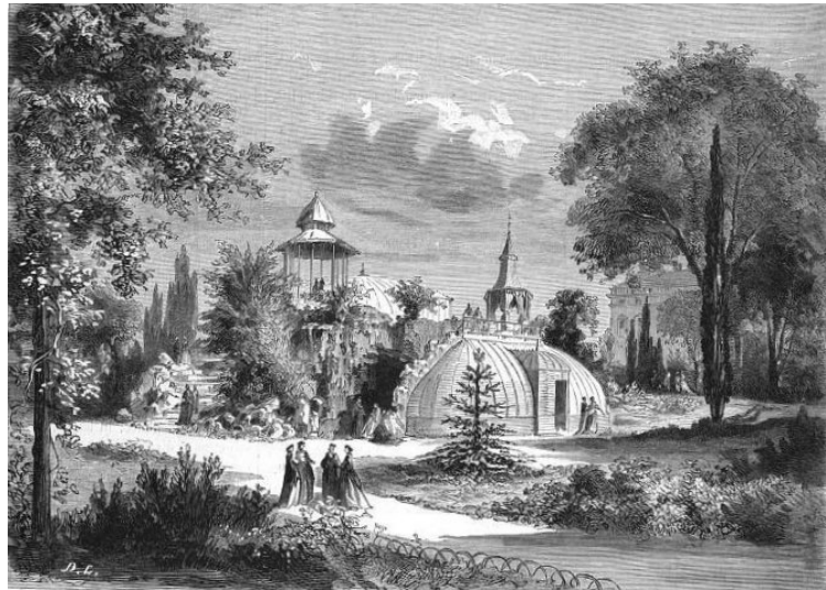
Figure 6.33 Grotto and belvedere of the aquarium, 1867 Exposition universelle . From L'exposition universelle de 1867, illustrée .
