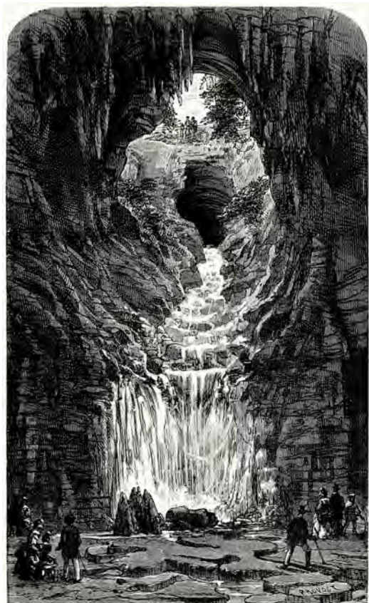
Figure 6.6 Alphand, Parc des Buttes-Chaumont, grotto . The cavern was a remnant of the former quarry, further shaped and structurally reinforced to form the grotto with cascade.
