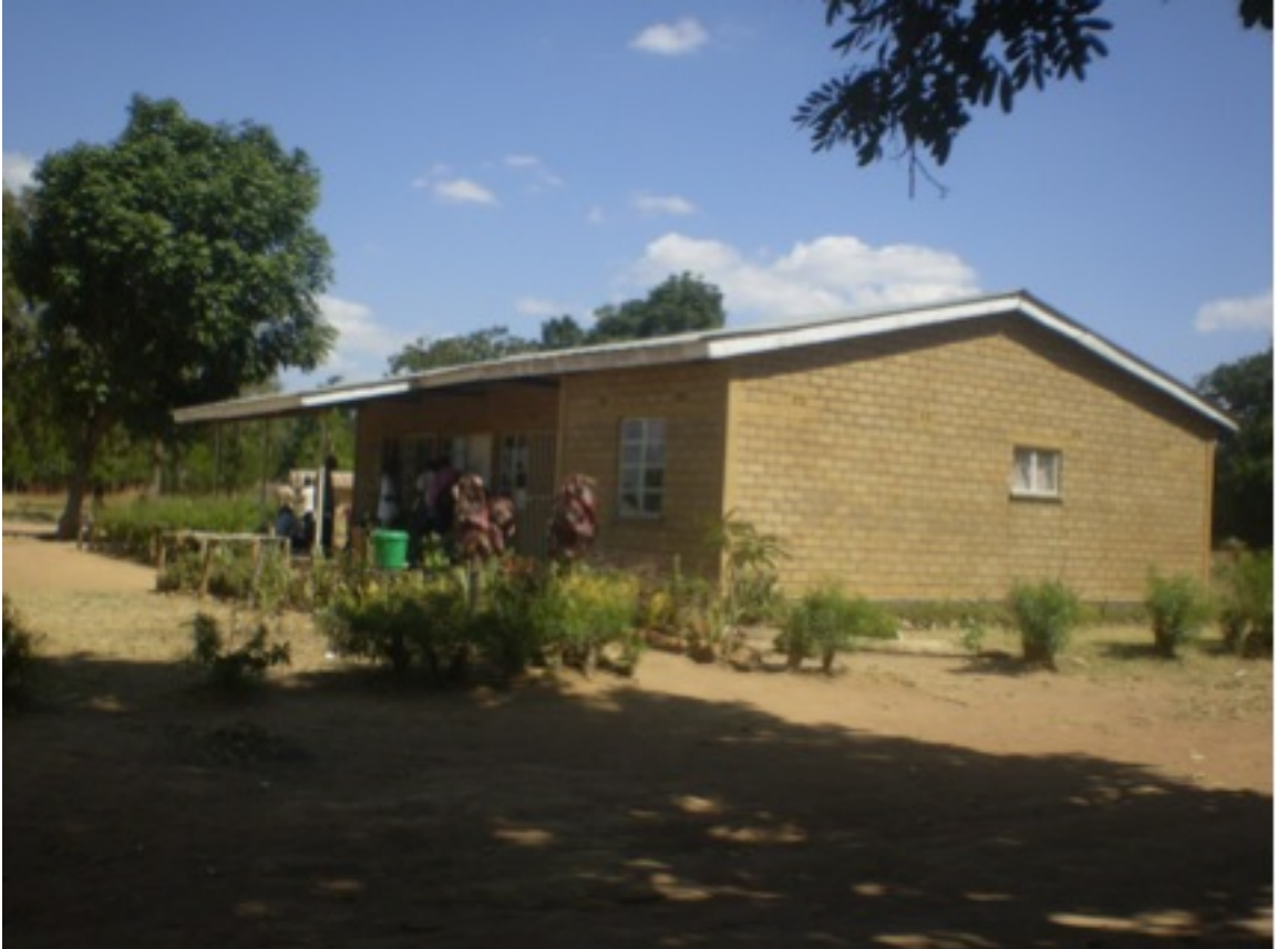
Figure 1.4: A teacher training college (TTC) building rented by a case study project. A ten-day training was held here in June 2008 (Photo: Author).
