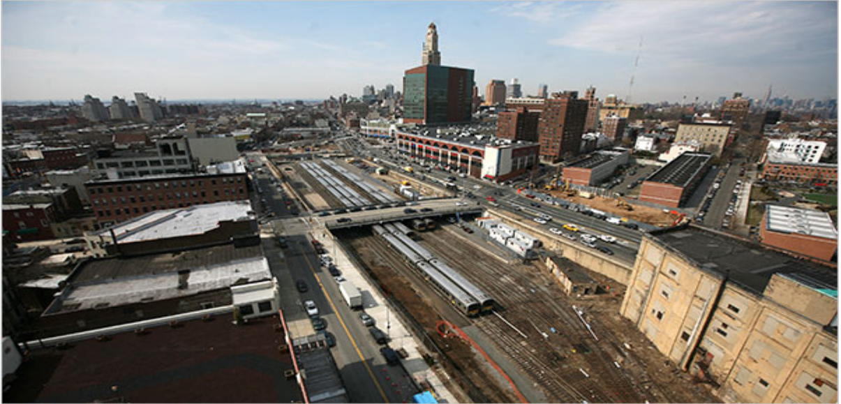
Figure 41. The proposed Atlantic Yards project would be located over a Long Island Rail Road train yard (Chang W. Lee/ New York Times ).
