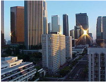
Figure 1. Los Angeles' Downtown Financial District. (City of Los Angeles).
