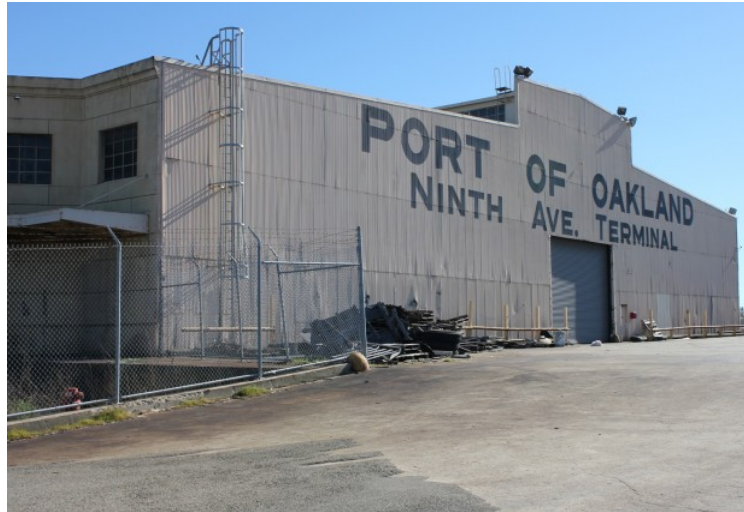
Figure 48. Most of the Ninth Avenue Terminal will be demolished under the current Oak to Ninth plan. It is currently being used as a cotton storage warehouse (Oakland Heritage Alliance).
