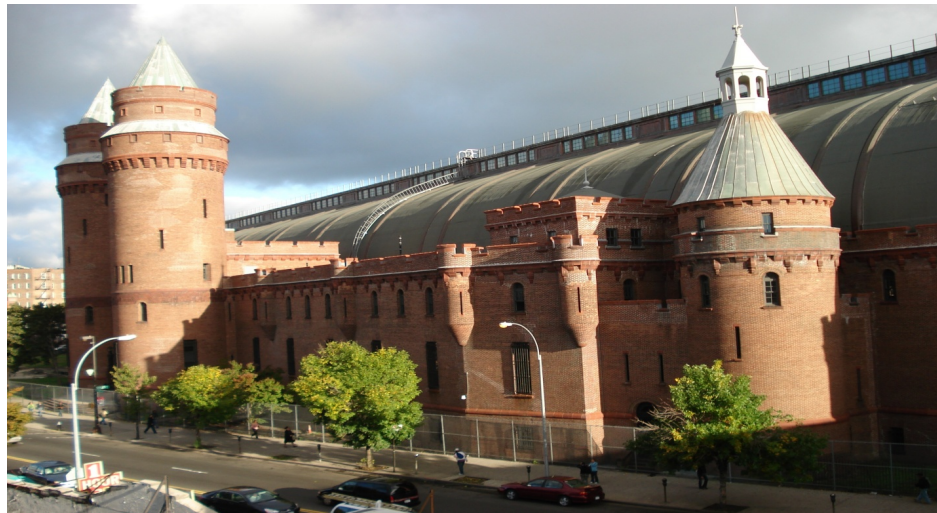
Figure 24. Since the early 1900s, the Kingsbridge Armory has served as a signature building in the Bronx (Cityland).
