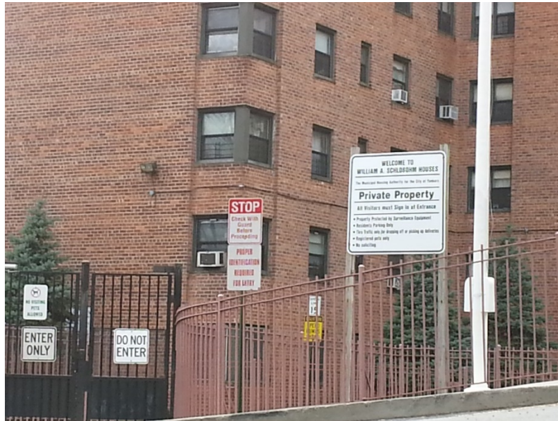
Figure 4. Schlobohm Houses, fencing and gates
