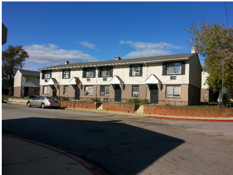
Figure 18. Eastport Terrace, barracks-style apartments
