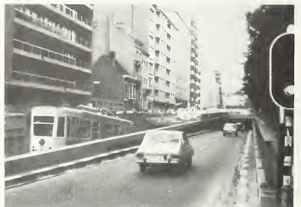
P-46 . Tunnel access ramp (Brussels)
