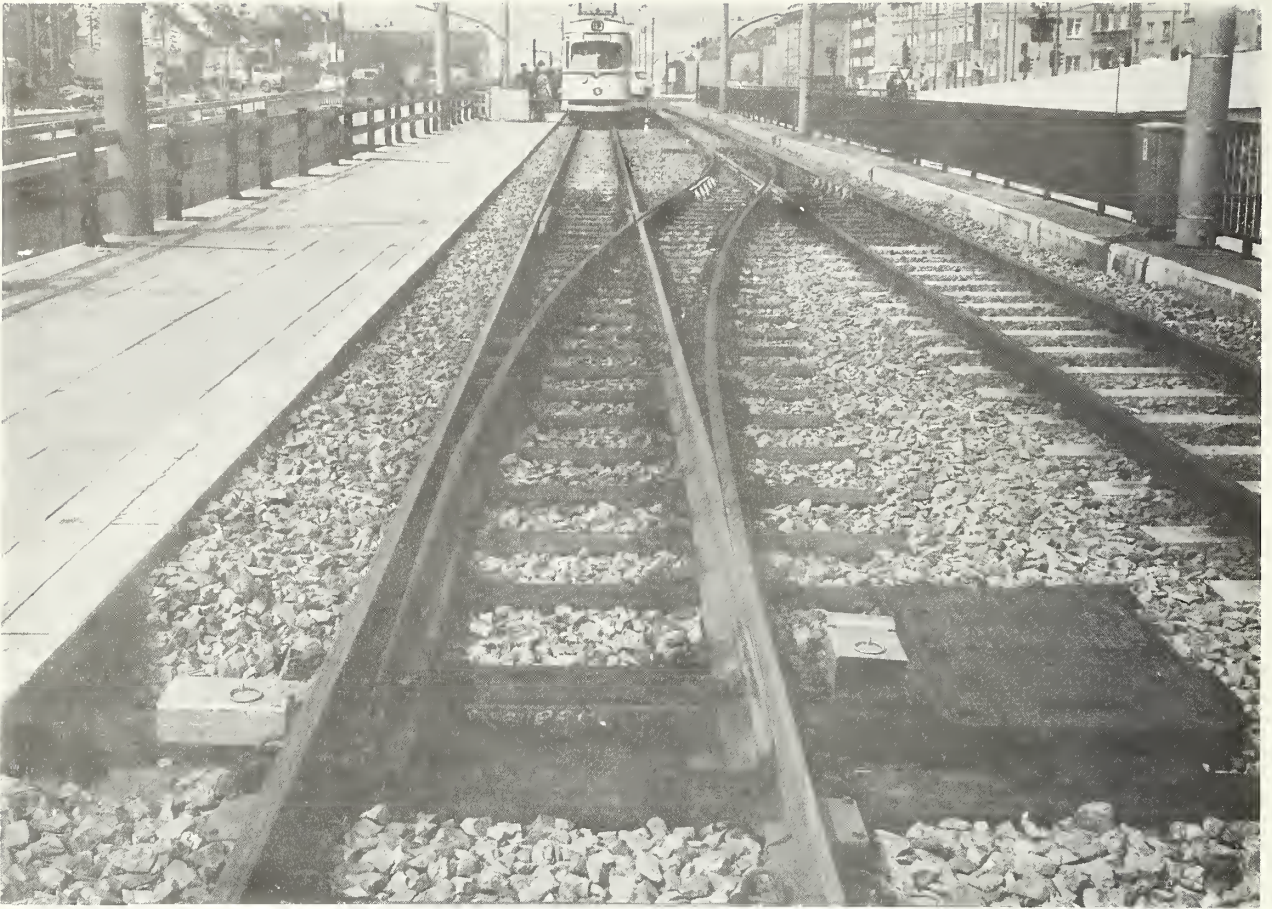
P-47. Modern switch with elastic points
