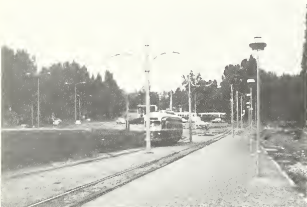
P-43 . Access to a viaduct; pedestrian walk on the right (Belgrade)
