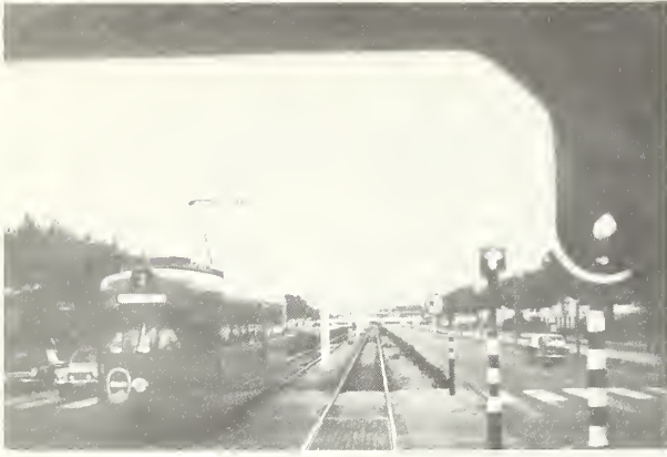
P-35 . Special signal ("T") for light rail (Rotterdam)
