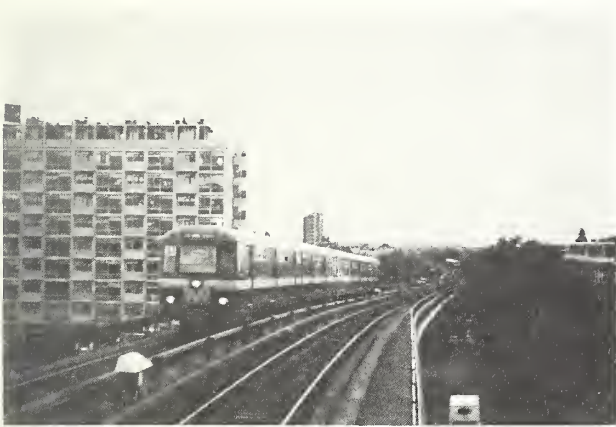
P-64. Elevated section of a new rapid transit line (Rotterdam)
