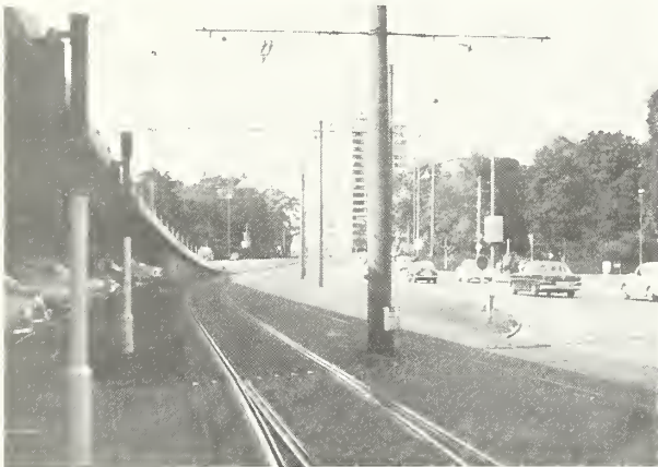
P-37 . Special switch with long points to allow switching prior to street crossing (Düsseldorf)
