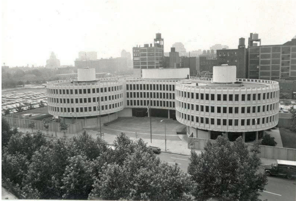
Figure 12. The Philadelphia Police Headquarters (1962) is Geddes, Brecher, Qualls, and Cunningham's most famous structure, the exterior of which consists of three-story tall structural precast wall panels. 89
