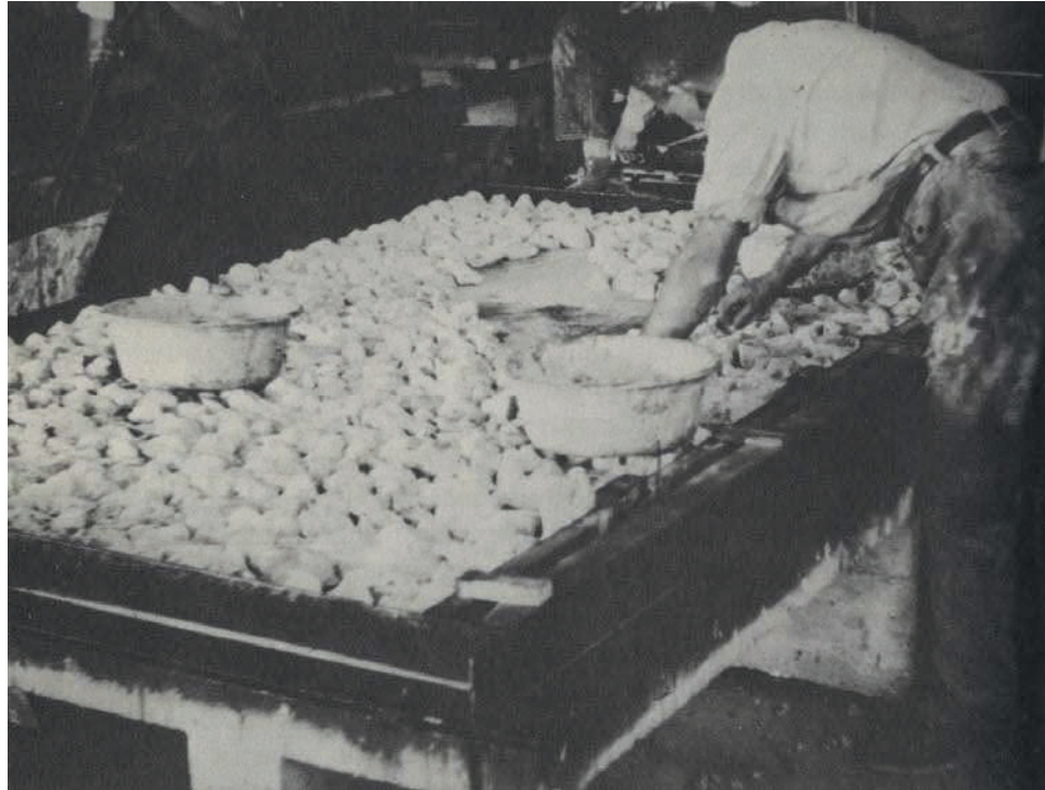
Figure 28. A precaster hand laying the facing aggregate in the formwork. 222
