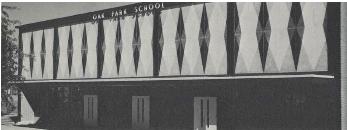
Figure 20. The Oak Park High School utilizes colored architectural precast wall panels on the school's façade. 109
