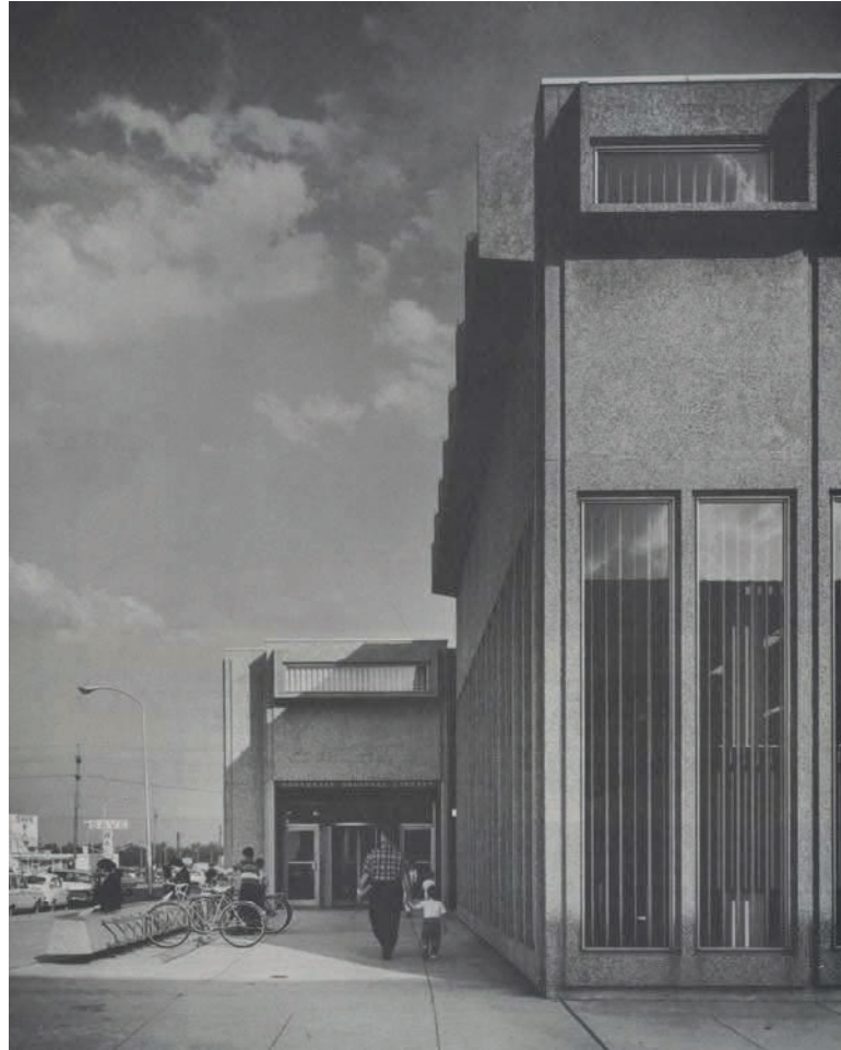
Figure 13. Geddes, Brecher, Qualls, and Cunningham’s design for the Northeast Regional Library in Philadelphia (1962) is clad with architectural precast wall panels, a detail of which is shown in this image. 92
