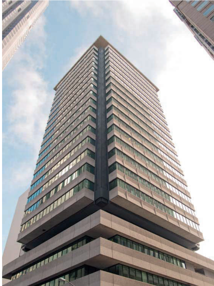
Figure 18. The elevations of the International Building in San Francisco, by Anshen and Allen (1961), are defined by alternating layers of glazing and precast undersills, whose reentrant corner design creates interesting shadows and depth. 102
