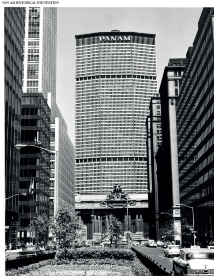
Figure 11. The Pan American Building in New York City (1962), designed by Walter Gropius and Pietro Belluschi, is clad with 9,000 story-high precast window units. 87
