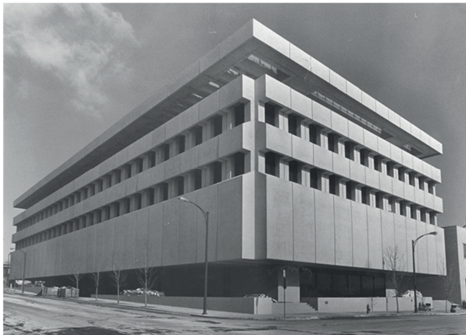
Figure 14. The Buffalo Evening News Building, designed by Edward Durell Stone and Associates (1973), is clad with massive architectural precast panels. 94
