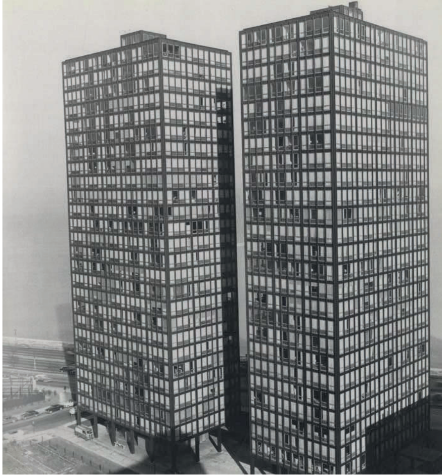
Figure 6. Lake Shore Drive Apartments by Mies van der Rohe (Chicago, 1948-1951). 61
