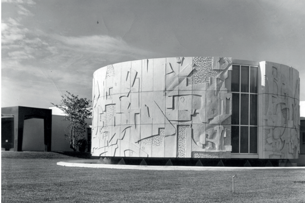
Figure 22. The panels used on the Miami Beach Public Library, designed by Herbert A. Mathes (1962), illustrate the expressive texture that could be achieved with architectural precast wall panels. 111
