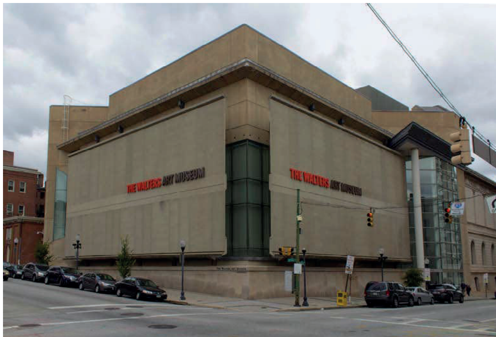
Figure 15. The precast panels of the Walters Art Museum addition in Baltimore, MD, designed by Shepley, Bulfinch, Richardson, and Abbot of Boston and Meyer, Ayres, and Saint of Baltimore (1974), form a brise soleil (photo by author).
