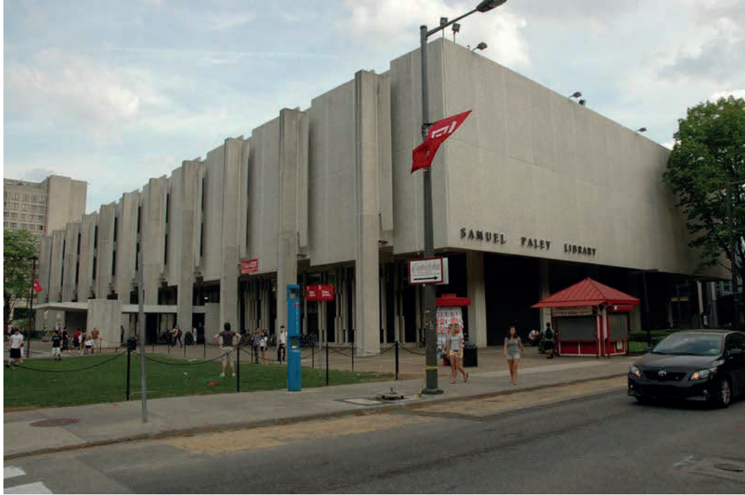
Figure 21. The Samuel Paley Library, designed by Nolen & Swinburne (1966), is clad with solid exposed aggregate panels. 110
