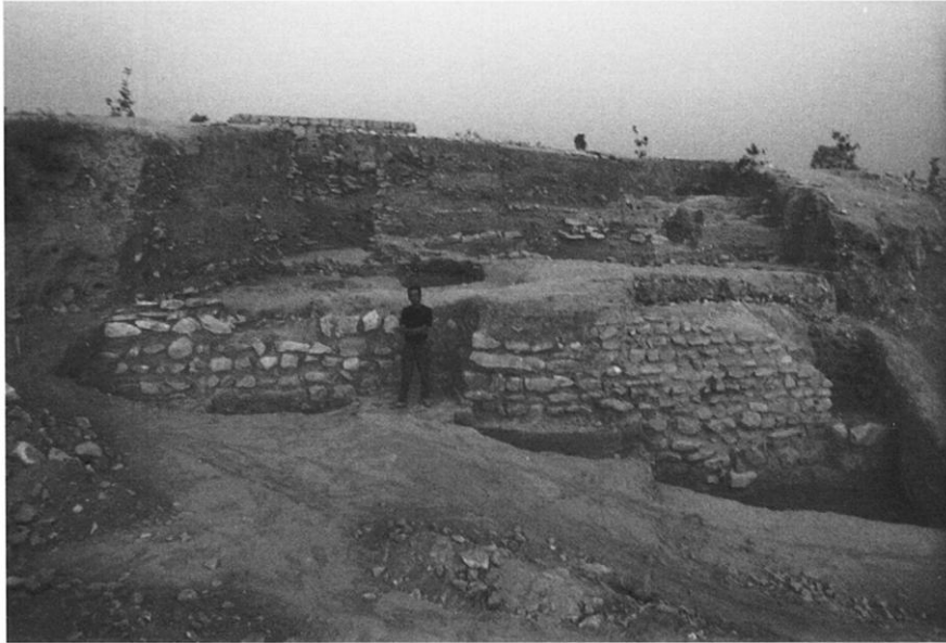
Fig. 7. Operation 1/6, phase B stone terrace platform
