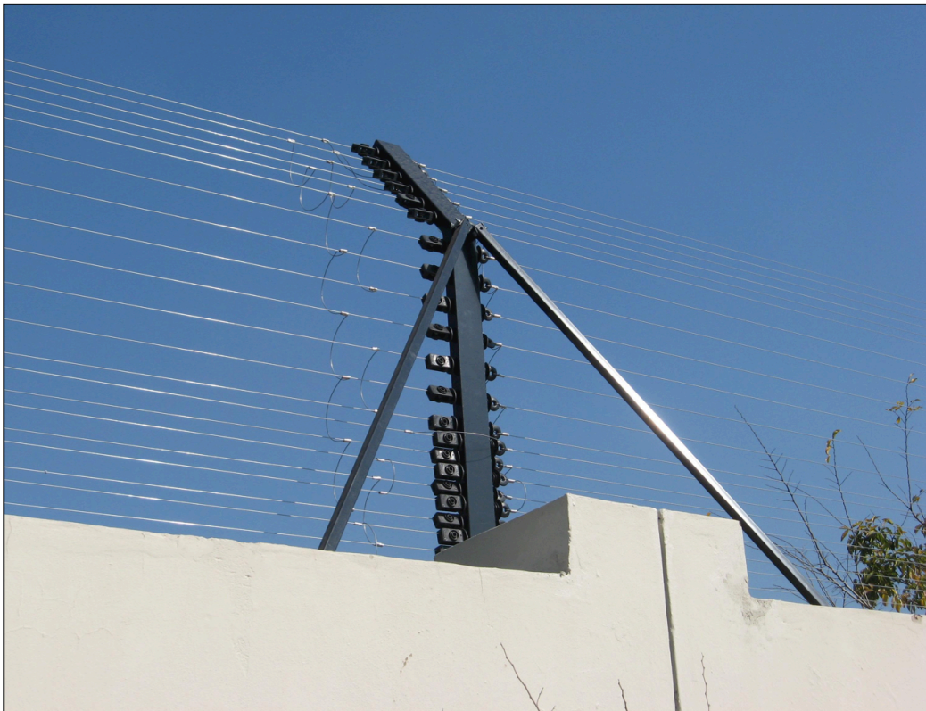
A close-up of rows of electric wire atop a concrete wall
