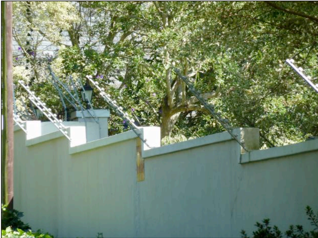
A typical concrete wall topped with multiple rows of electric wire
