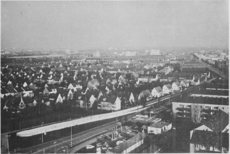
Figure 23. LRT transition from surface to tunnel in Hannover, W. Germany
