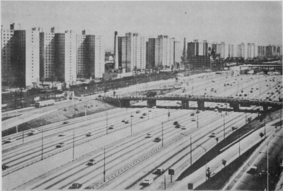
Figure 2. Incompatible land uses: 18 highway lanes adjacent to residences (Chicago)
