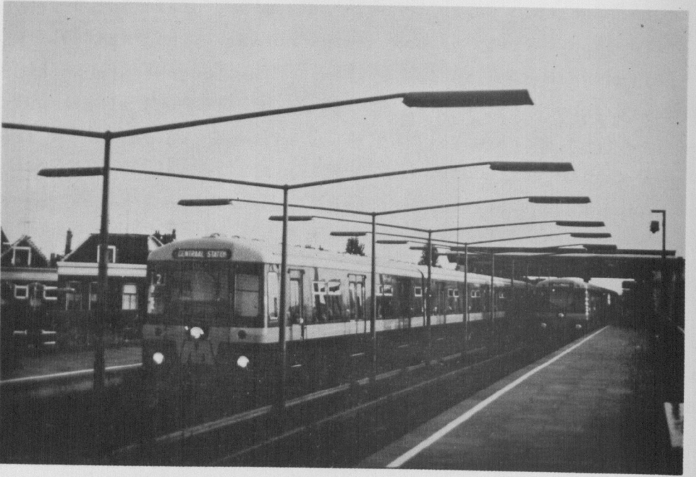
Figure 39. Aerial station on the Rotterdam Metro system
