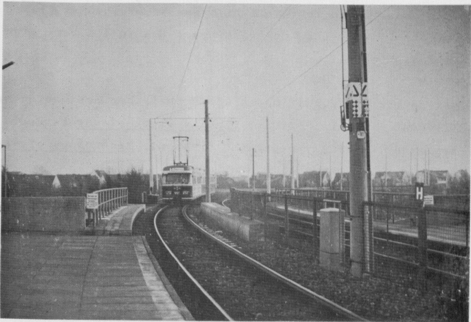
Figure 26. LRT line to a new suburban residential development (Bremen, W. Germany)
