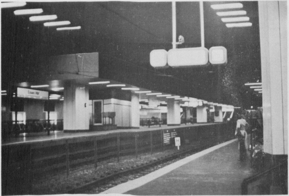
Figure 24. LRT underground station in downtown Hannover
