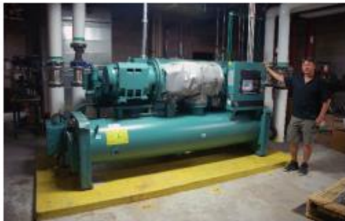
Figure 1: 100-ton water-cooled chiller. Water-cooled chillers use cooling towers to reject heat through evaporation.
