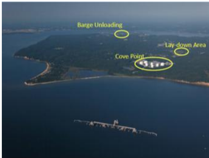
Figure 3.5: Current Cove Point LNG Import Facility
