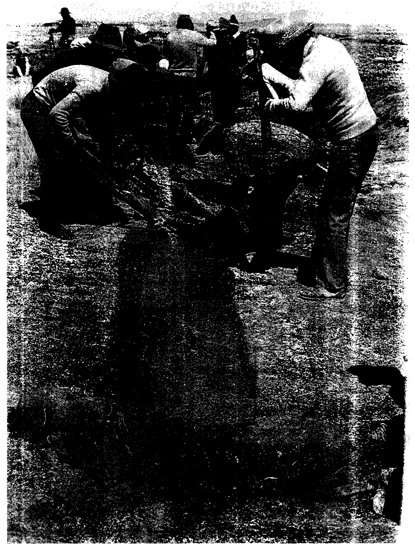
6.16. The use of chakitaqllas for construction of the retaining walls of experimental raised fields.
