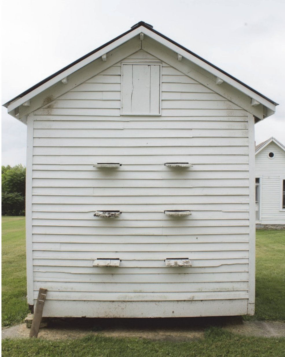
Figure 25 Vernon Bee House Rear Elevation. Photo by Author.
