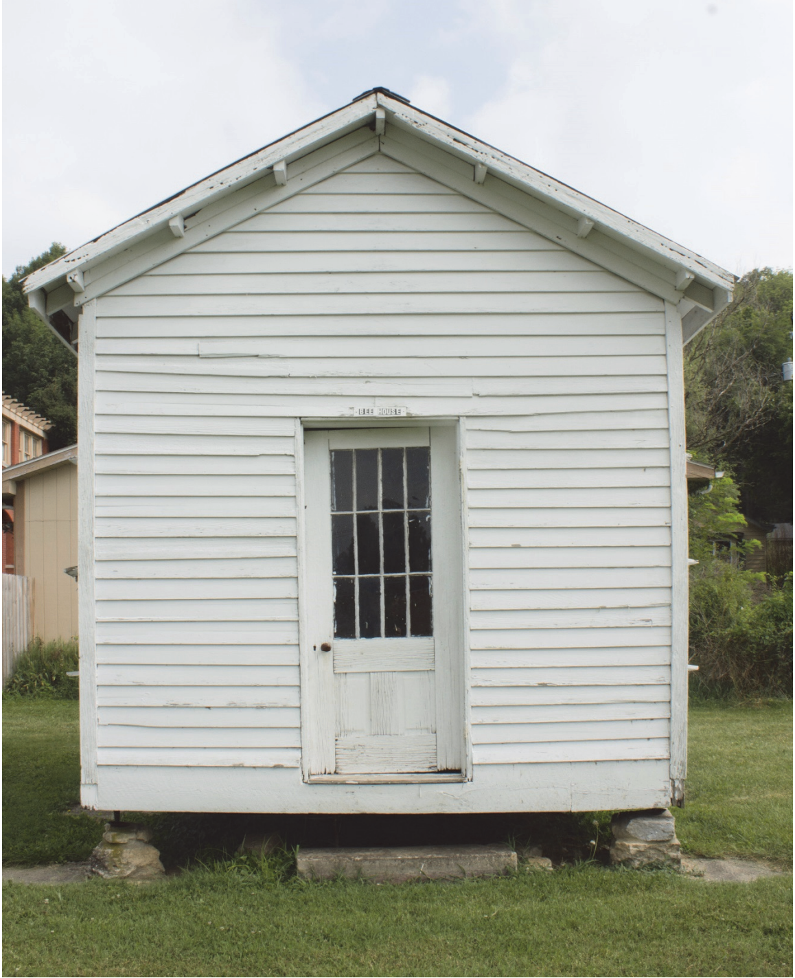
Figure 21 Vernon Bee House in Pearl Park, Madison, Indiana, door allowed beekeeper to enter house. Photo by Author.
