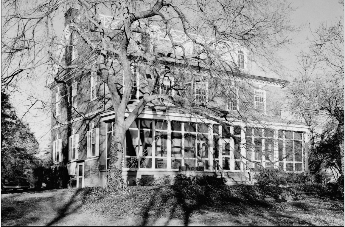
Figure 5.2. PA-1628-1 Front (South) Side. Photograph by Theodore F. Dillon, 1958. Courtesy of Library of Congress, Historic American Building Survey.
