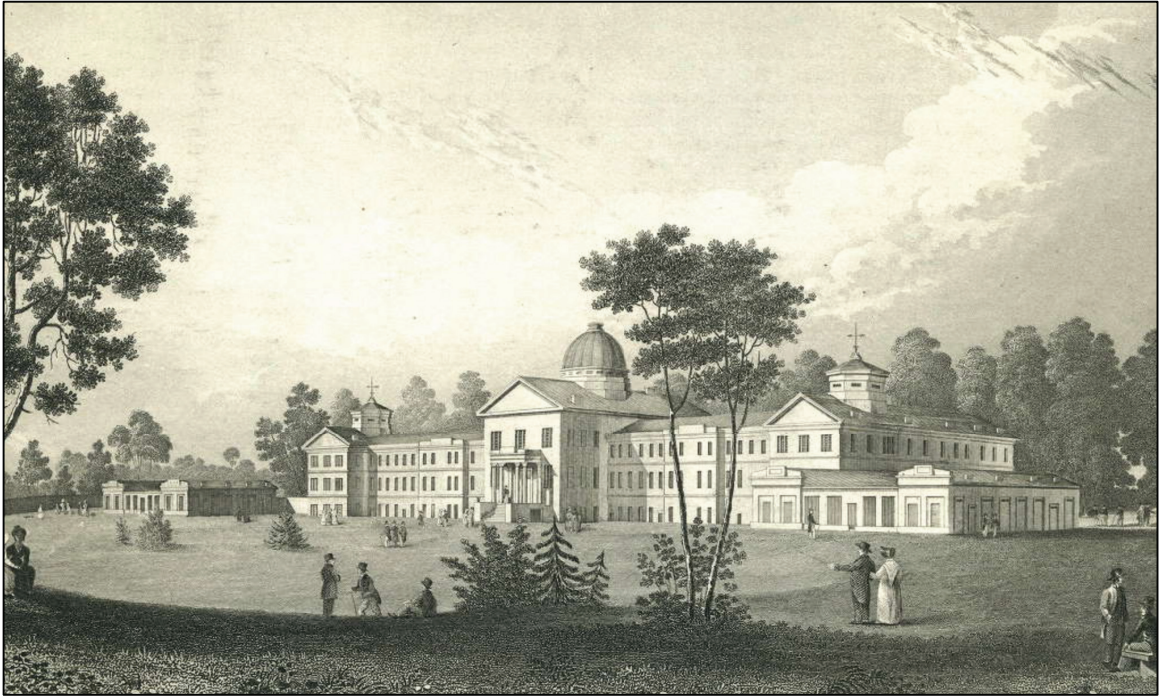
Figure 4.1. Pennsylvania Hospital for the Insane at 44 th and Market Streets. It was designed by Isaac Holden, complete in 1841, and demolished in 1959. Lithograph by W. Mason, artist, and W.E. Tucker, engraver, c. 1845. Courtesy of the Free Library of Philadelphia.
