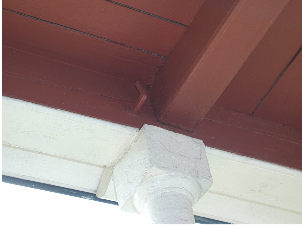
Figure 15. Present day photograph detailing the beading of the beams. Image credit MCH.
