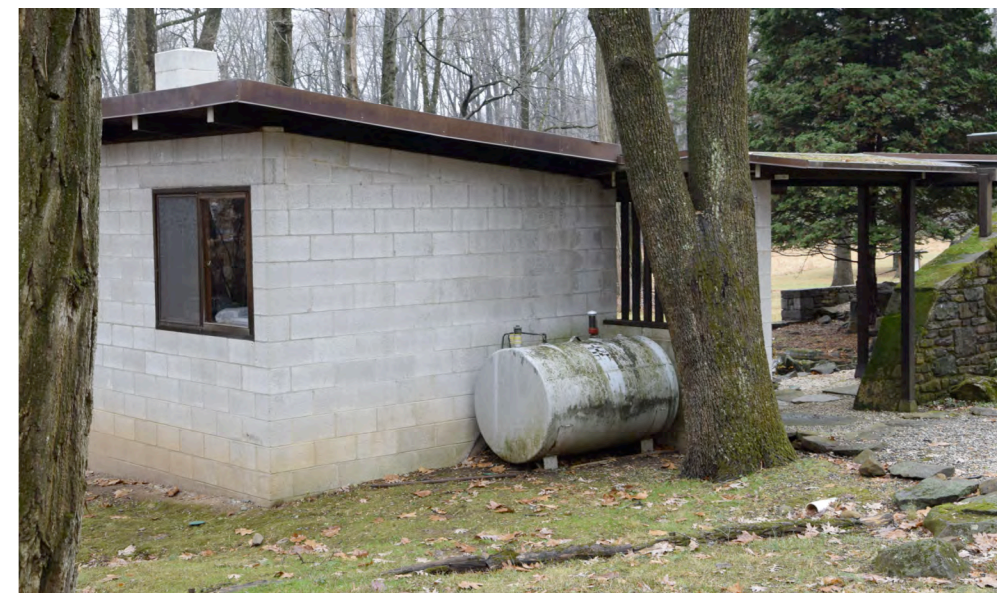
Cloister exterior view from the northeast
