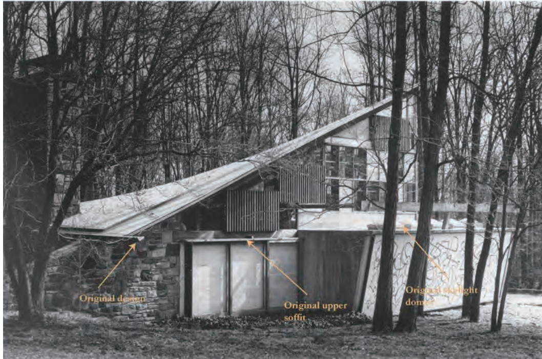
Fig. 4.1: West elevation view. Date: Notice the original gutters, the upper soffit in the sliding window, and the skylight domes. In addition, the concrete floor of the terrace as originally built. Source: George Nakashima Woodworker SA, Ltd. Archives.
