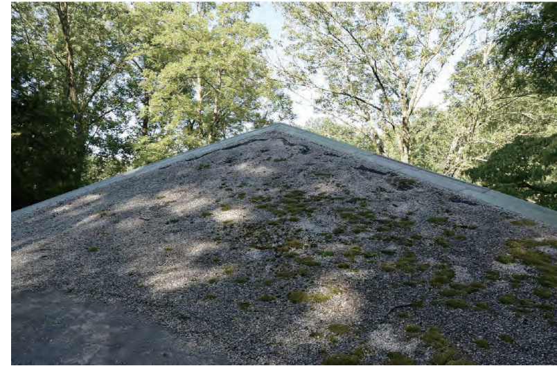
Closer view of the upper section
