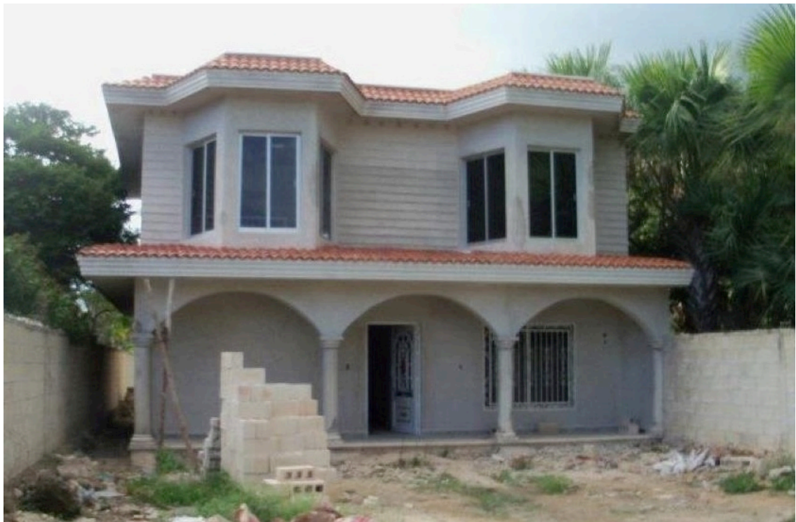
Figure 3.3. Concrete molded to look like horizontal siding (2 nd floor). Oxkutzcab, Yucatán. December 2011. Photograph by Alberto Pérez Rendón. Used with kind permission from Mariel Caamal.
