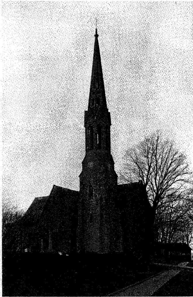
Figure 19: Second Congregational Church 139 East Putnam Avenue, Greenwich, CT 1856-58
