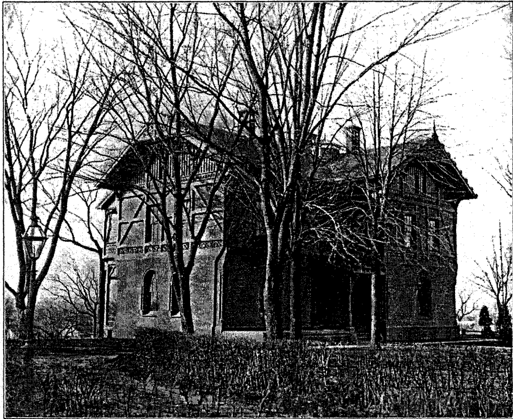
Figure 30: Murray-Vermilye House Englewood, NJ c. 1861
