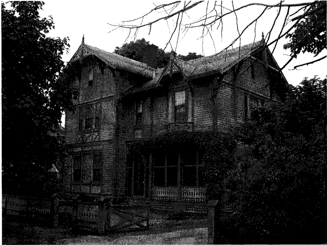
Figure 21: William A. Booth Residence
