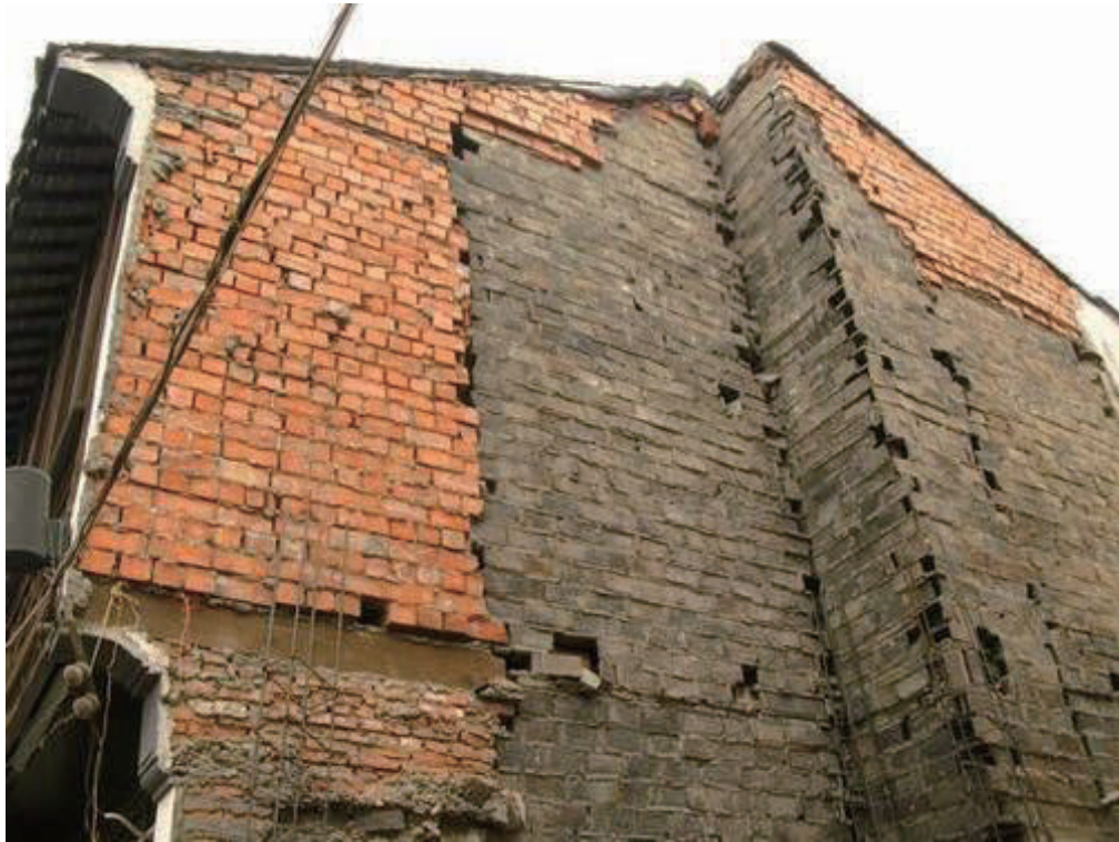
Figure 2.1.2 A historical building on Pingjiang Rd (平江路), Soochow, originally built with grey bricks, renovated with red bricks (Photo by Wenwen Xia)
