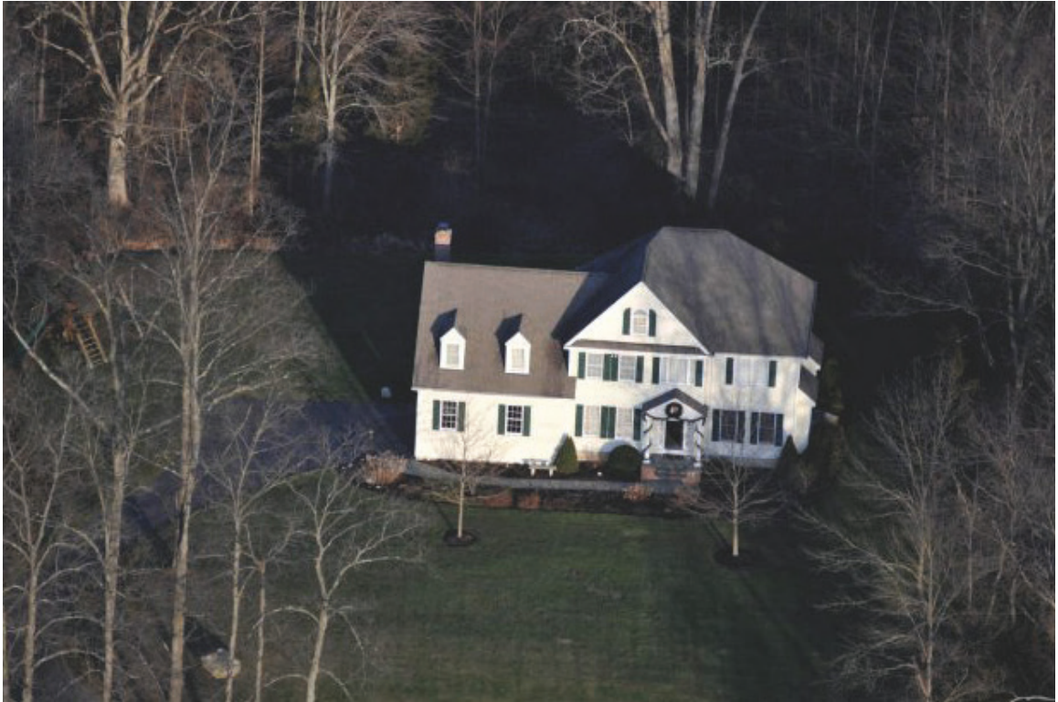
FIGURE 3.2: Aerial image of the residence shared by Adam Lanza and his mother prior to its demolition on March 23, 2015. The intention to recast the site as a tabula rasa, to “return the land to a natural state” and eliminate its associations with violence, becomes clearer in recognition of the context of both the house and the Sandy Hook Elementary School on vast properties bordered by woods.
