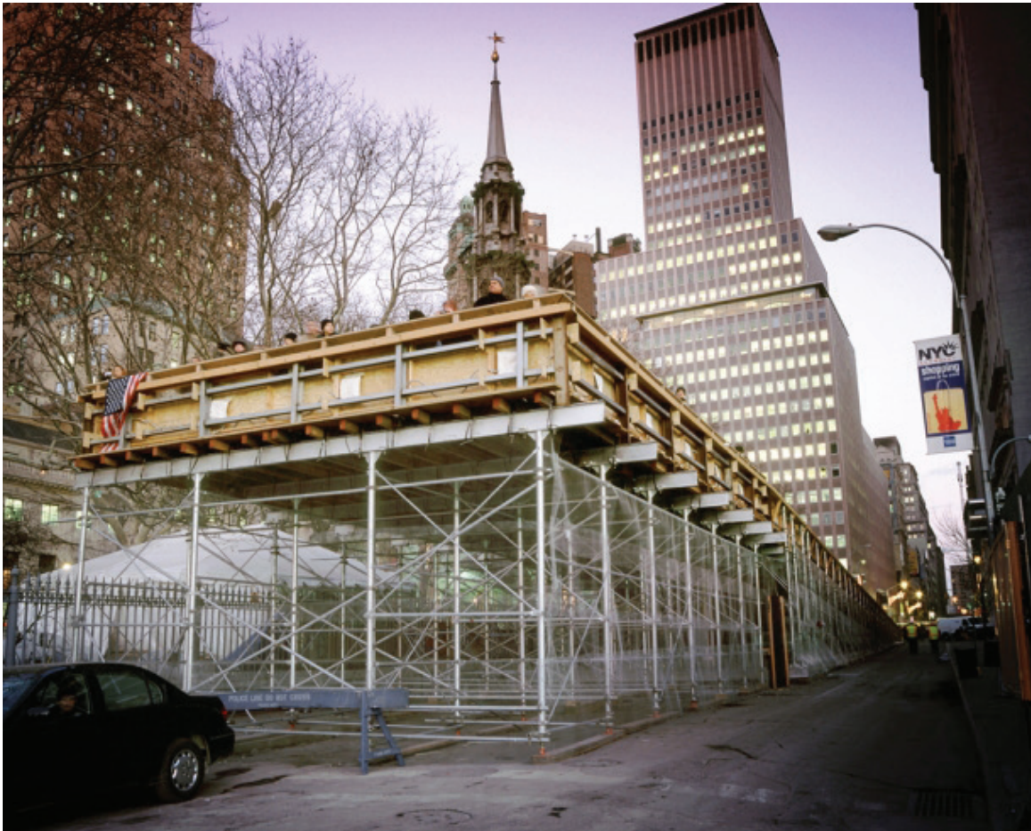
FIGURE 2.3: Though diller scofidio + renfro employed “metal scaffolding, plywood, and rough decking” 31 to de-emphasize the fact of the platform as a designed work of architecture, the rhythmic, regular spacing of materials and the careful logic of smooth interior surfaces versus spaced and framed exterior surfaces points to the structure as a designed rather than impromptu work. For this and other reasons, the platform was viewed as “ghoulish” by families of victims.
