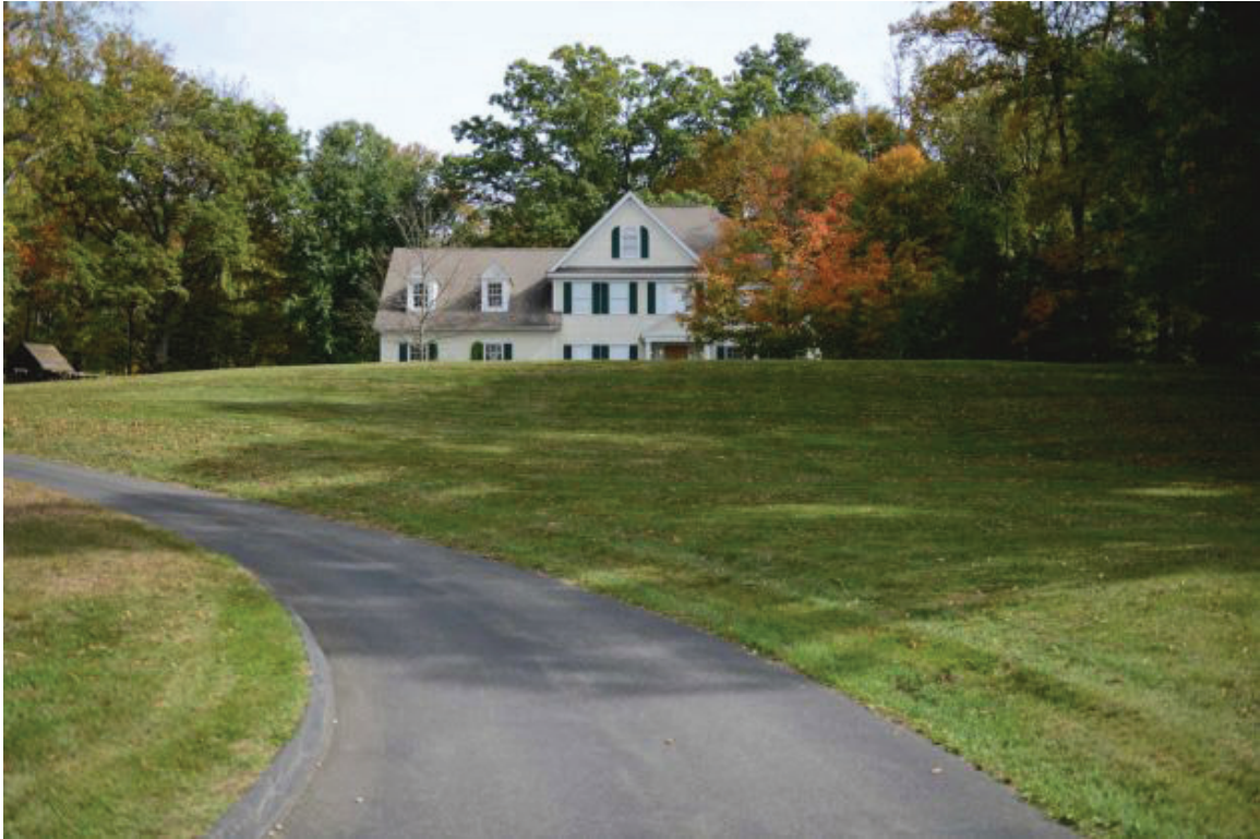
FIGURE 3.3: The residence shared by Adam Lanza and his mother prior to its demolition on March 23, 2015. The intention to recast the site as a tabula rasa, to “return the land to a natural state” and eliminate its associations with violence, becomes clearer in recognition of the context of both the house and the Sandy Hook Elementary School on vast properties bordered by woods.
