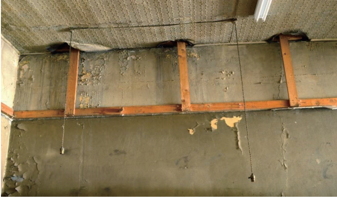
Figure 3.30 Historic wiring for single suspended bulbs (Author 2014).
