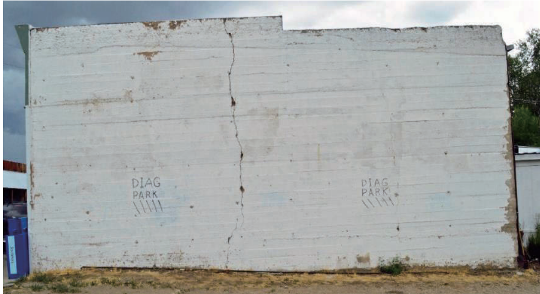
Figure 3.5 Exposed west wall (Author 2014).
