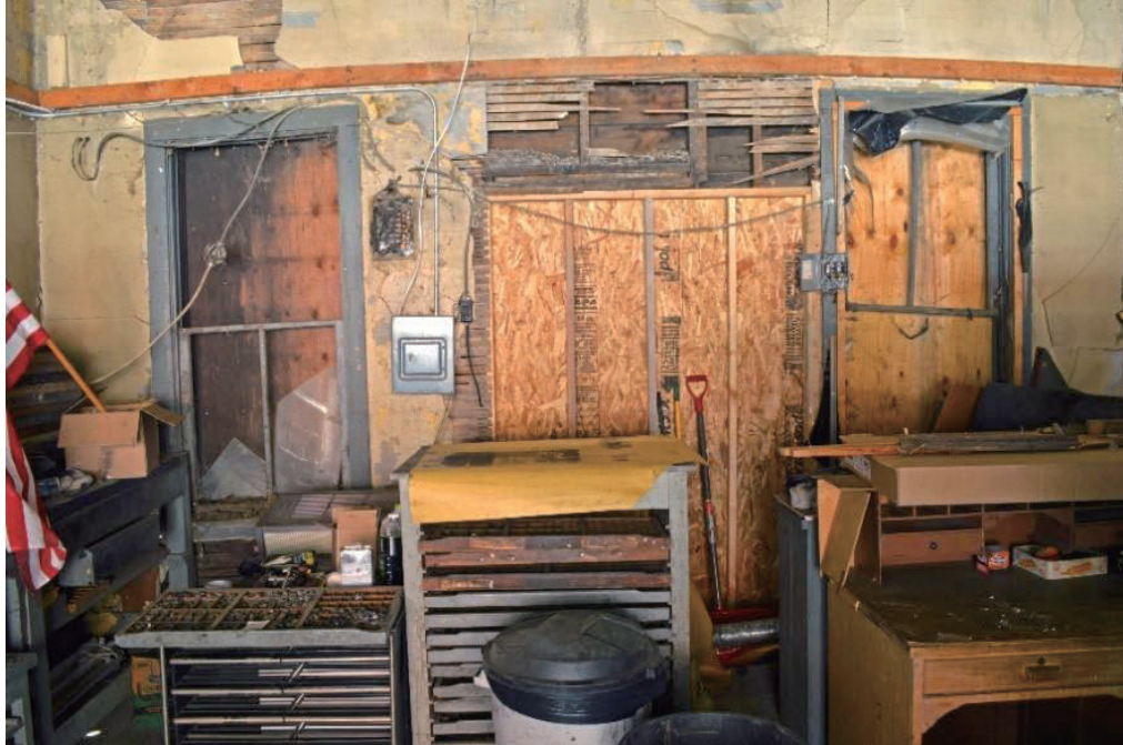
Figure 3.12 Interior view of rear wall showing entryway and windows (Author 2014).
