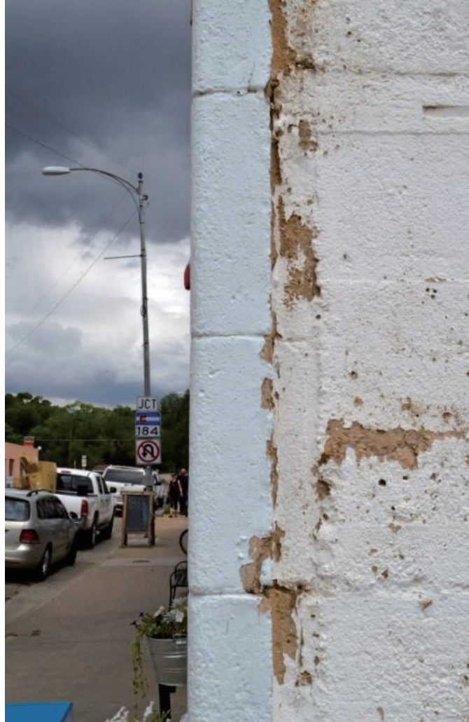
Figure 3.16 Decorative concrete block attached to west sidewall (Author 2014).
