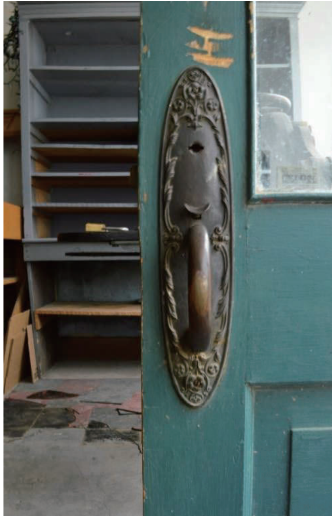
Figure 3.17 Decorative thumb latch front door handle (Author 2014).
