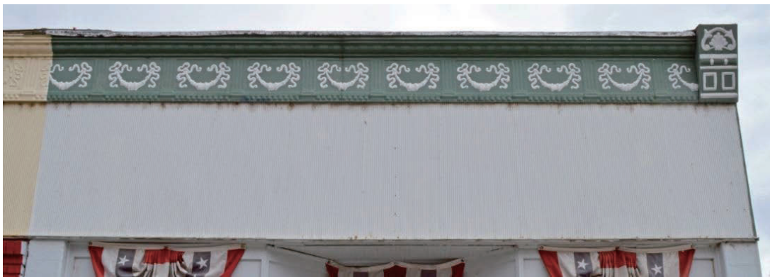
Figure 3.18 Decorative pressed metal cornice and architrave (Author 2014).
