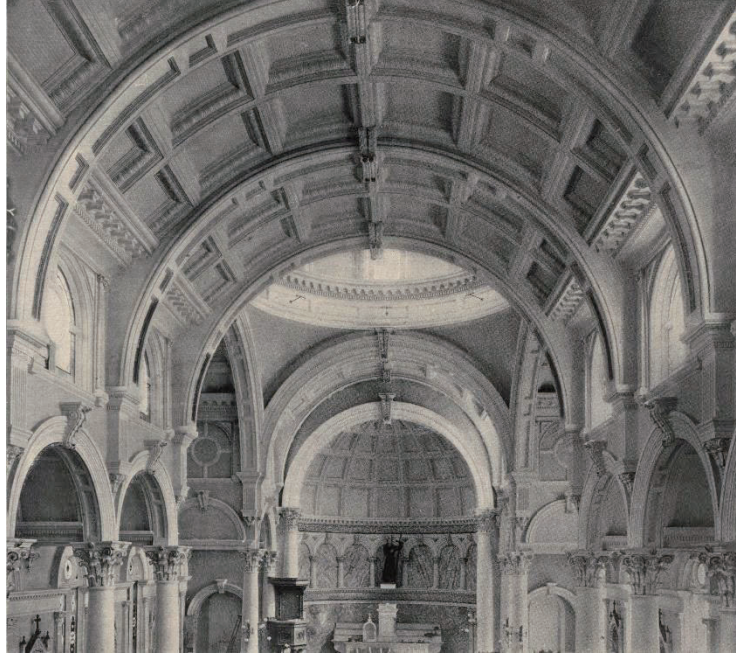
Figure 4.30 Metal ceiling of St. Leonard's Church in Boston (Northrop Coburn & Dodge Co., 45). 81
