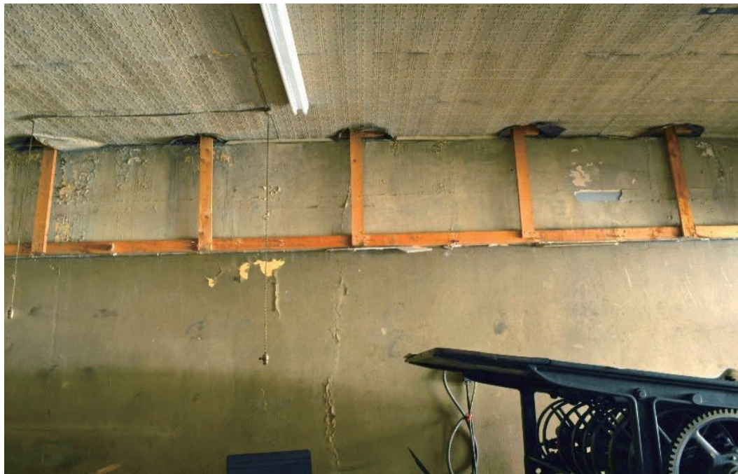
Figure 3.24 Remaining drop ceiling framing showing the cut pressed metal ceiling (Author 2014).
