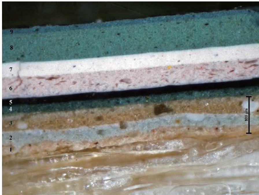
Figure 6.2 Comparison between the finish stratigraphies of the panel (MTT 03, top) middle rail (MTT 02, bottom) and of the front door (Author 2015).
