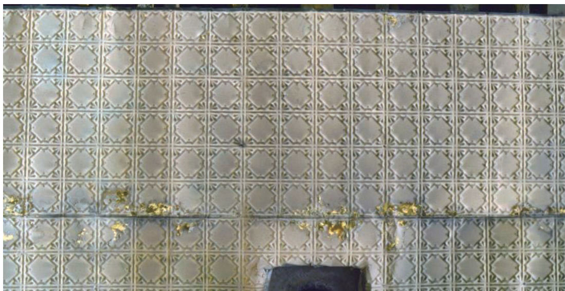
Figure 3.22 Pattern of the pressed metal ceiling (Author 2014).
