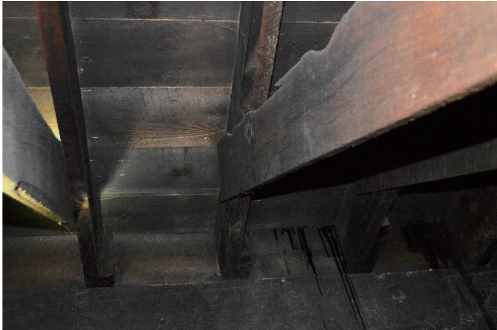
Figure 3.11 View of the roofing system showing rafters and decking boards (Author 2014). 4
