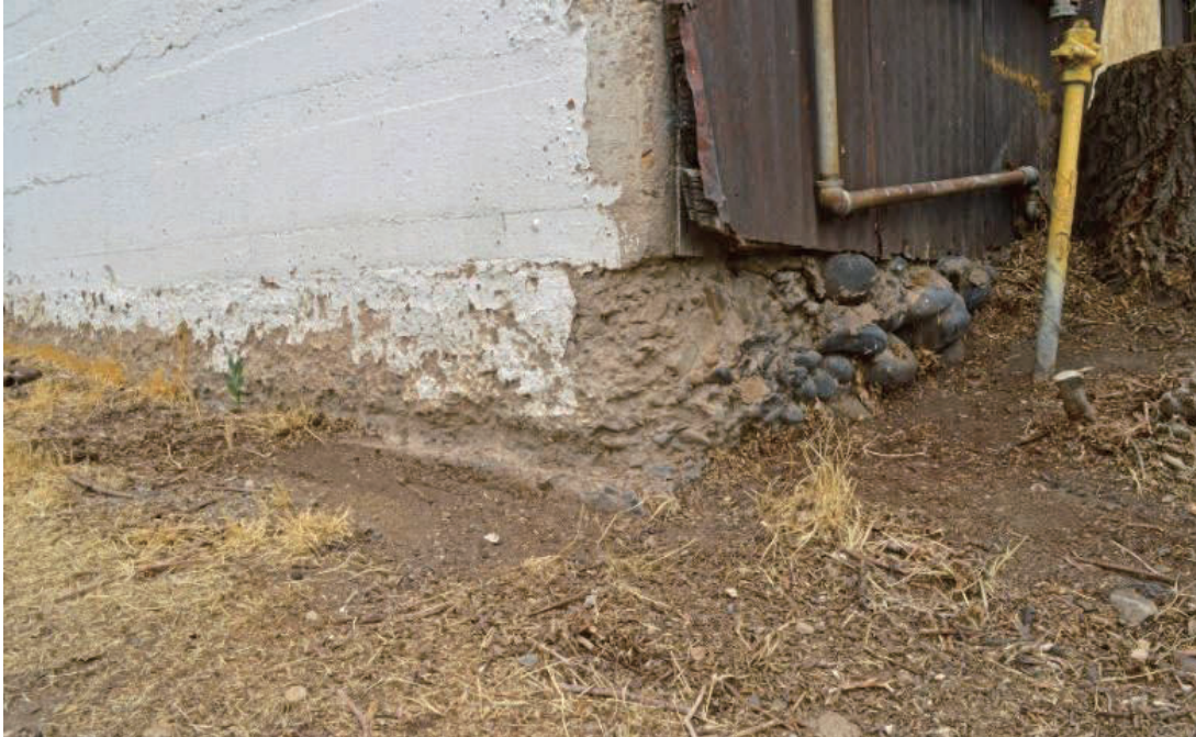
Figure 3.4 Two-part foundation with west supporting wall above (Author 2014). 1
