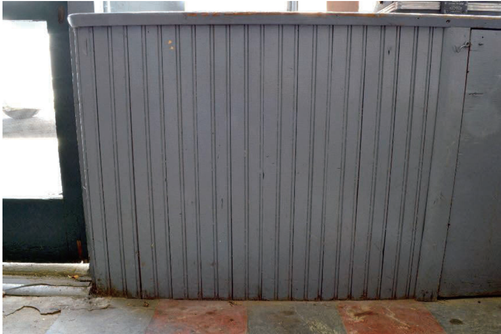
Figure 3.20 Front of eastern window display area (Author 2014).
