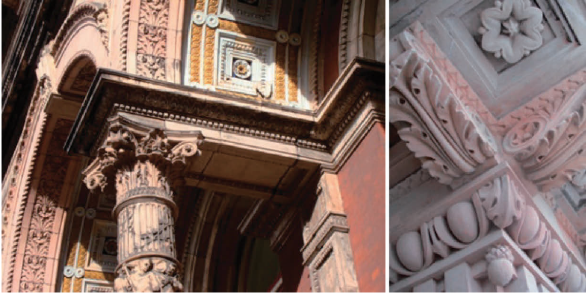
Figure 3: Before and after cleaning of the Henry Cole Wing in London, 2010. This building was cleaned by using a chemical gel formulation, and then rinsed with steam. Source: www.buildingconservation.com
