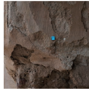
TUMA_14 Dark orange voussoir with pencilled white joints and black border
