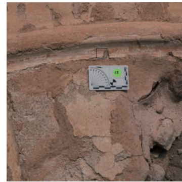
TUMA_13 Yellow and white, both extrados molding and scored joint
