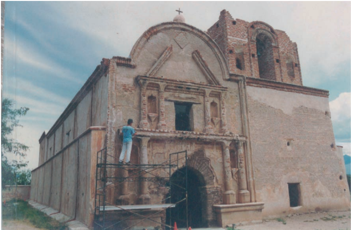
Figure 5.2: 1992 treatment to facade
