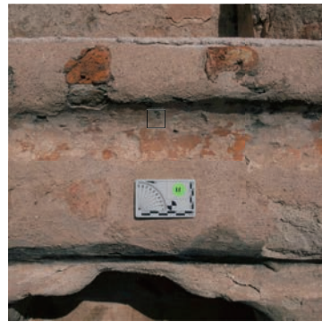
TUMA_11 Yellow, 1st scratch coat ~1/8", 2nd scratch coat ~1/4", 3rd coat limewash, 4th coat color
