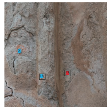
TUMA_18 Repair to TUMA_15 TUMA_19 Original finish
