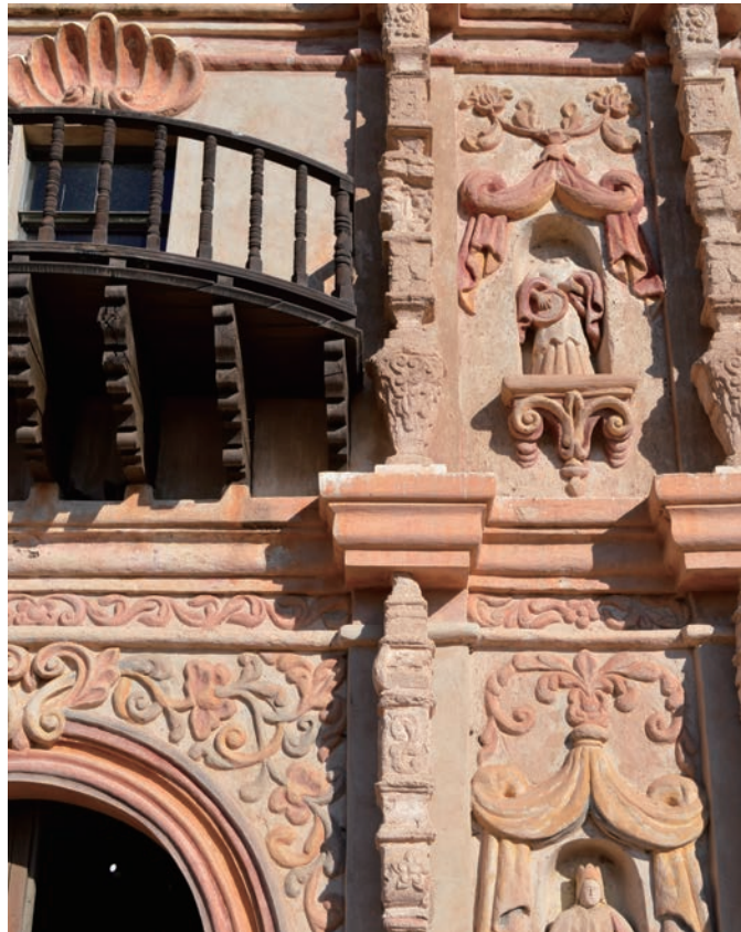
Figure 2.2: Detail of San Xavier del Bac façade
