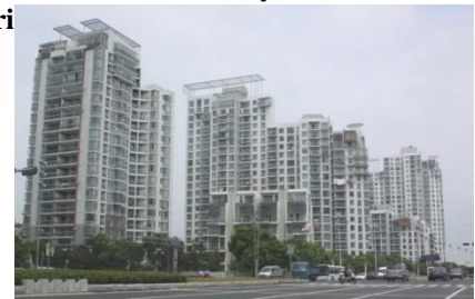
Figure 5.3: Housings in SIP I Source: Ibid.
