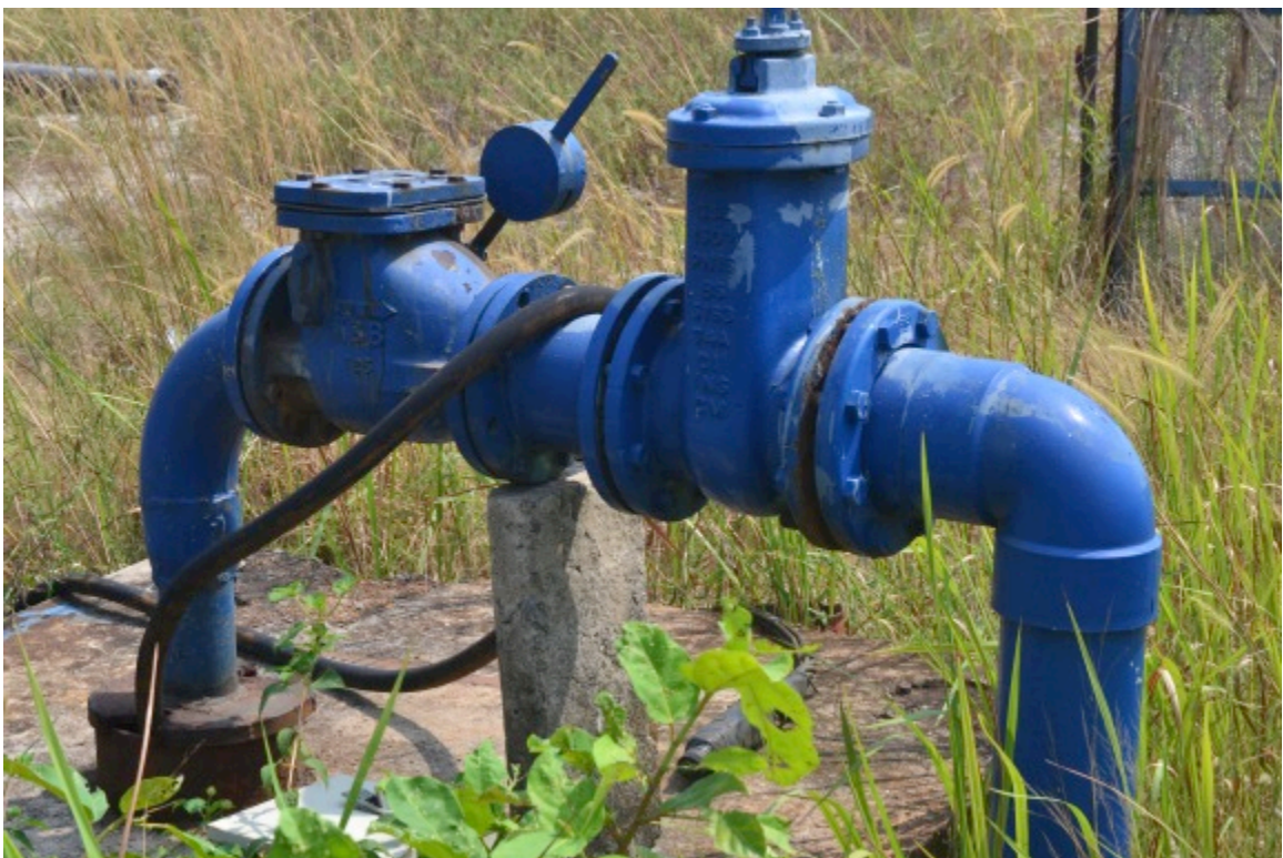
Figure 17: Borehole at Lekki Waterworks
