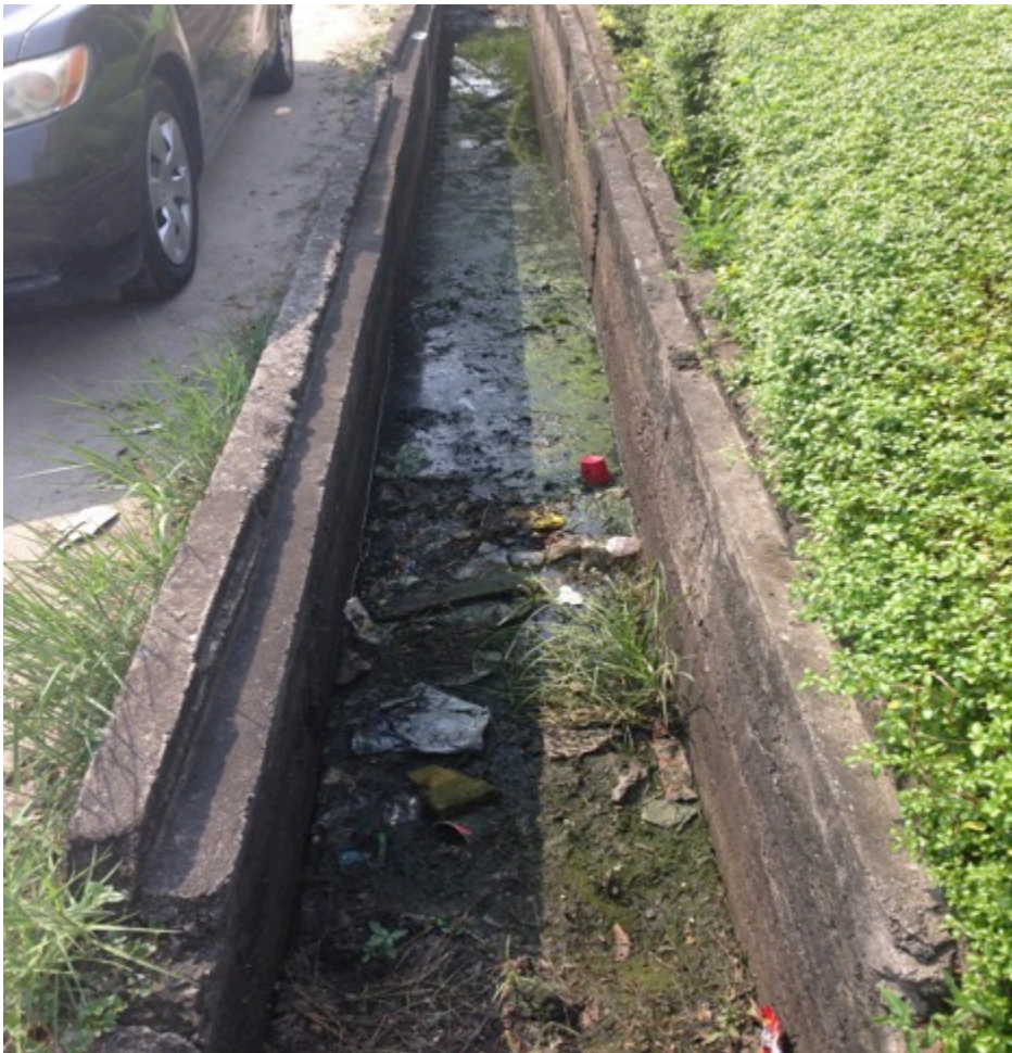
Figure 10: Blocked Drainage
