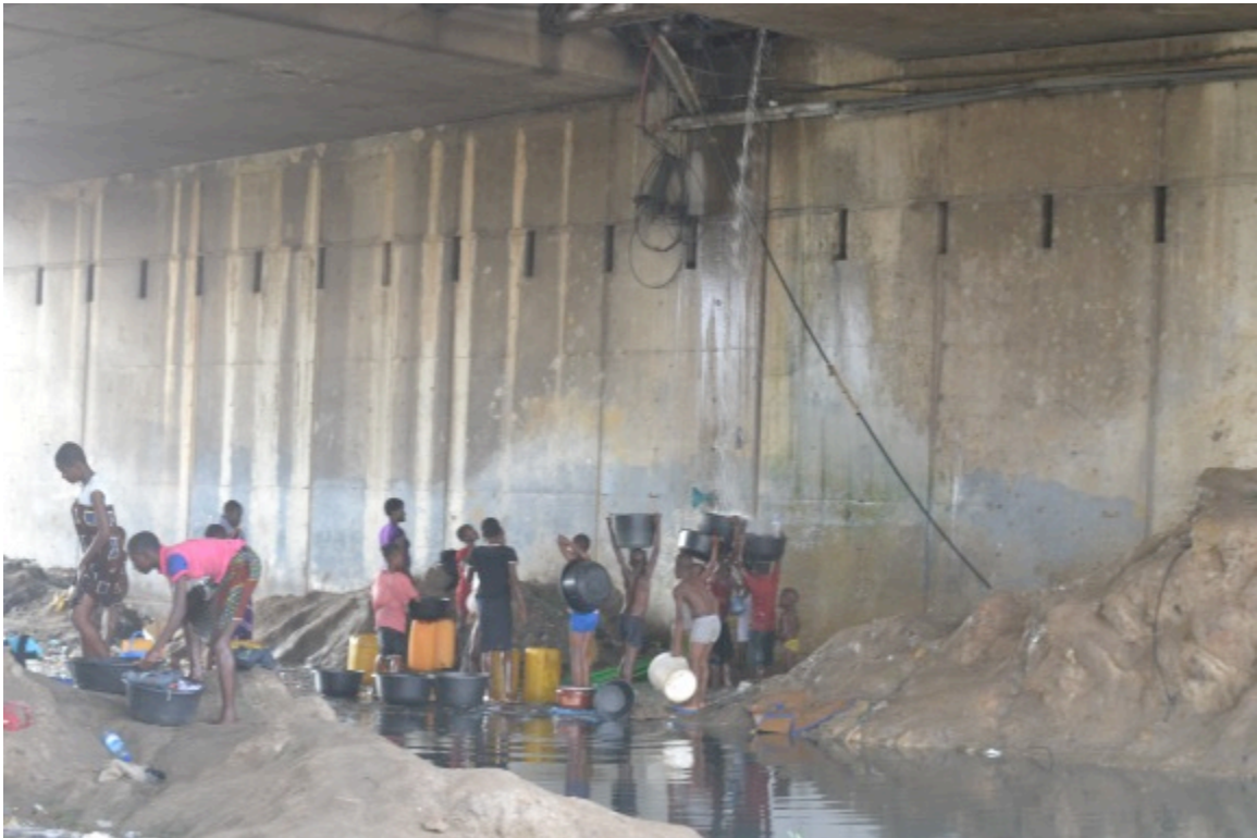
Figure 13: Water Leaking From Burst Pipe
