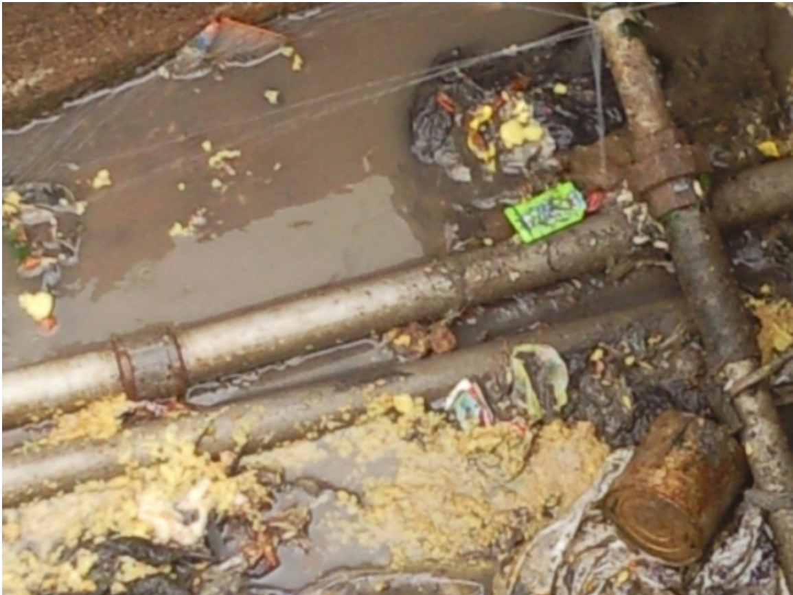
Figure 5: Water Pipes in Sewers
