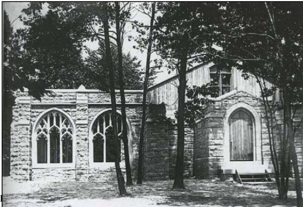
Figure 37. An early image of the chapel with only two completed bays of the Cloister and a temporary wooden roof (Swiggart, 67).
