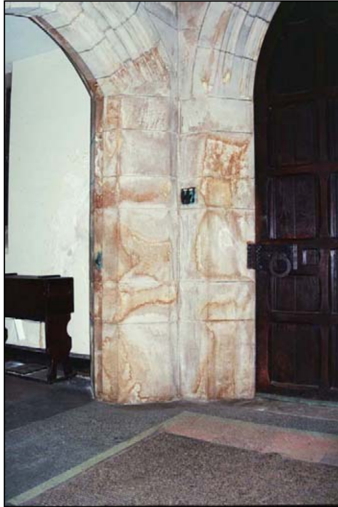
Figure 52. Limestone panels located to the north of the library entrance.
