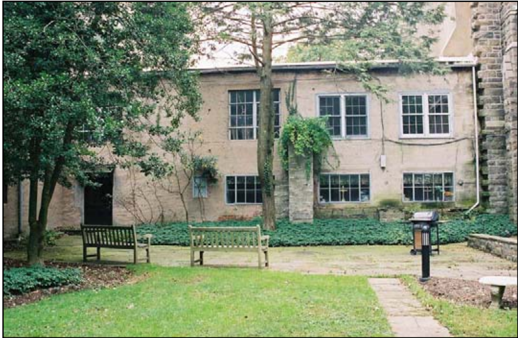
Figure 26. North façade of Patriot's Hall with stucco finish over brick, containing basement entrance.
