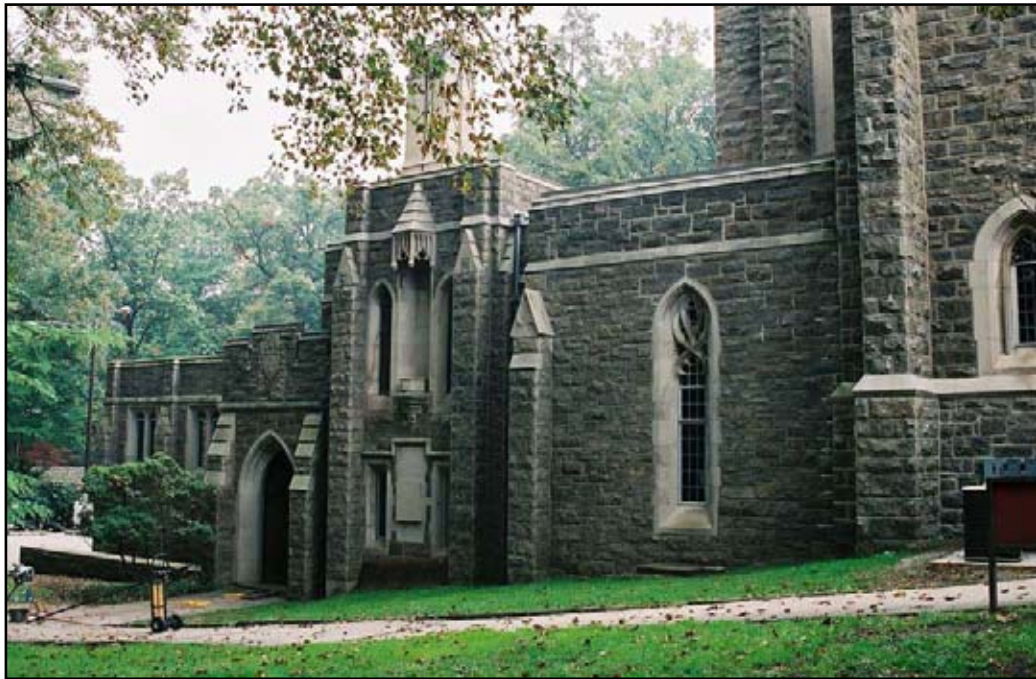
Figure 18. West façade of the Bishop White Library.
