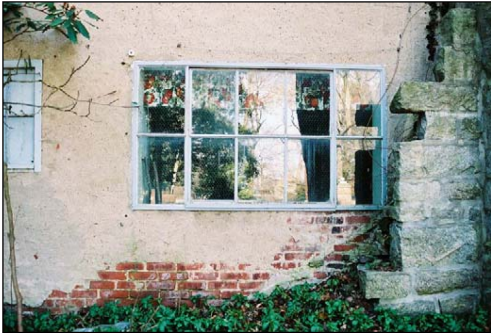
Figure 27. Toothed granite masonry intended to be extended upon the completion of Patriot's Hall.
