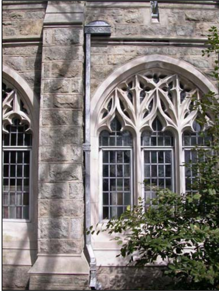
Figure 62. Example of the lead downspouts found within the Cloister.
