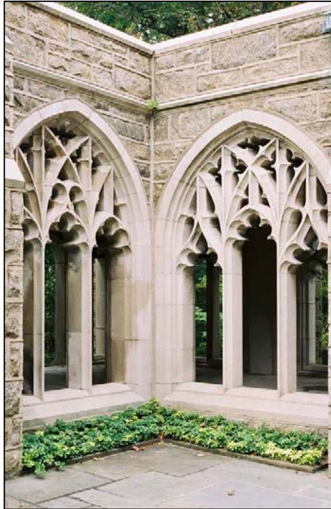
Figure 15. The design of each adjacent bay is distinct from its neighbor.
