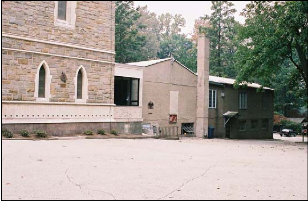
Figure 32. The museum addition extending north from the carillon.
