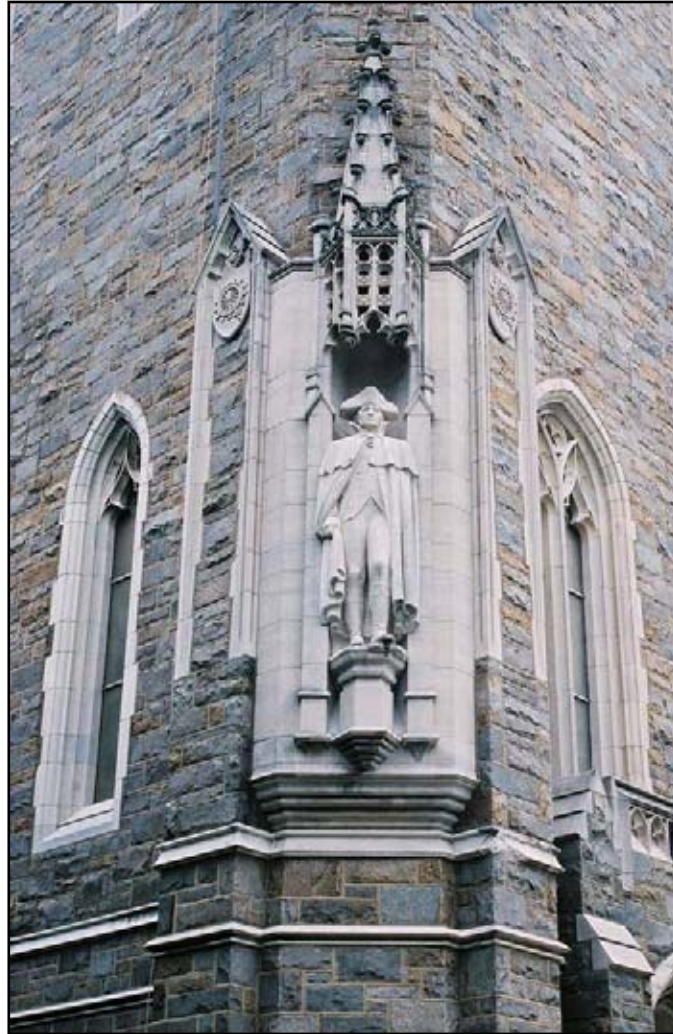
Figure 29. Limestone statuary located on the southwest corner of the tower.
