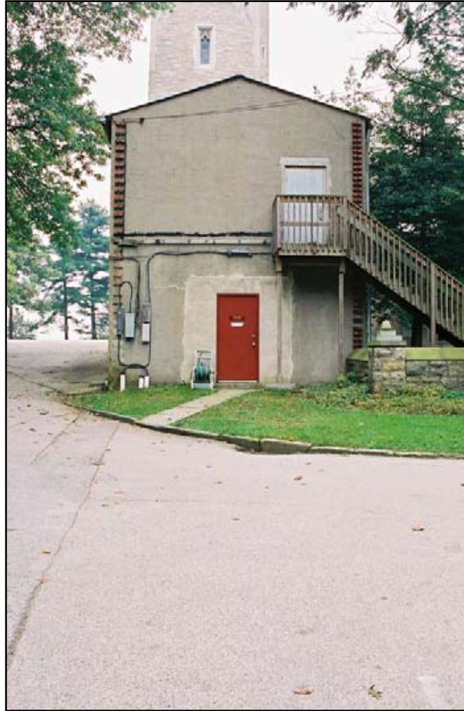
Figure 33. North façade of the addition.
