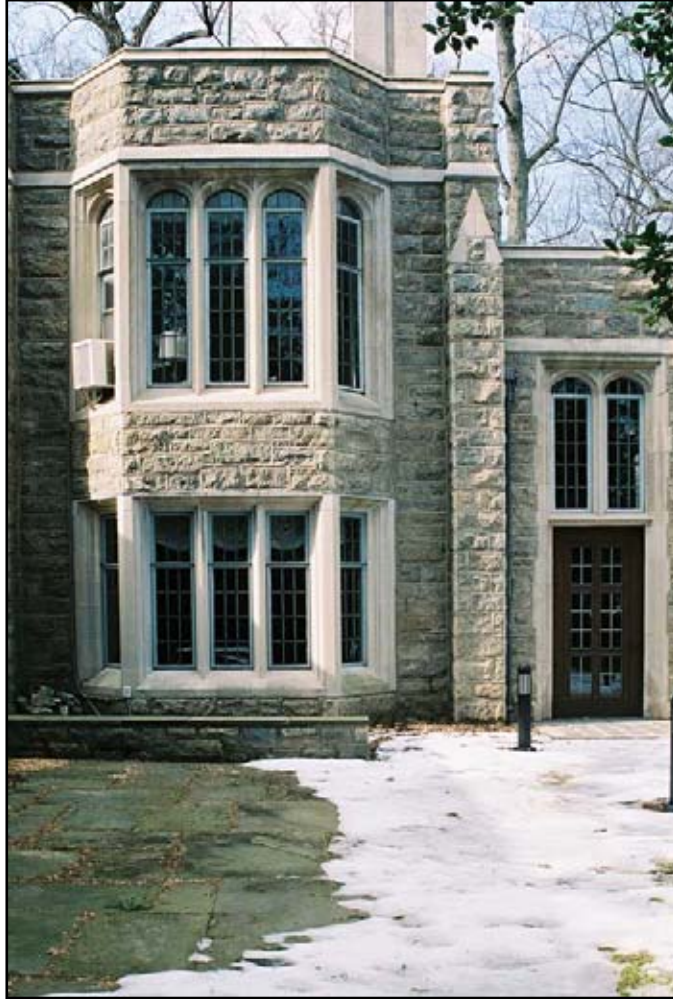
Figure 23. Bay window of the dining room.
