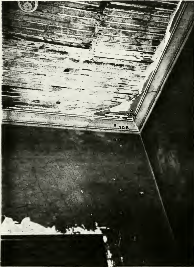
Figure 120: Photograph of Sample 30 Area: Connecting Room to Mrs. Lockwood's Room
