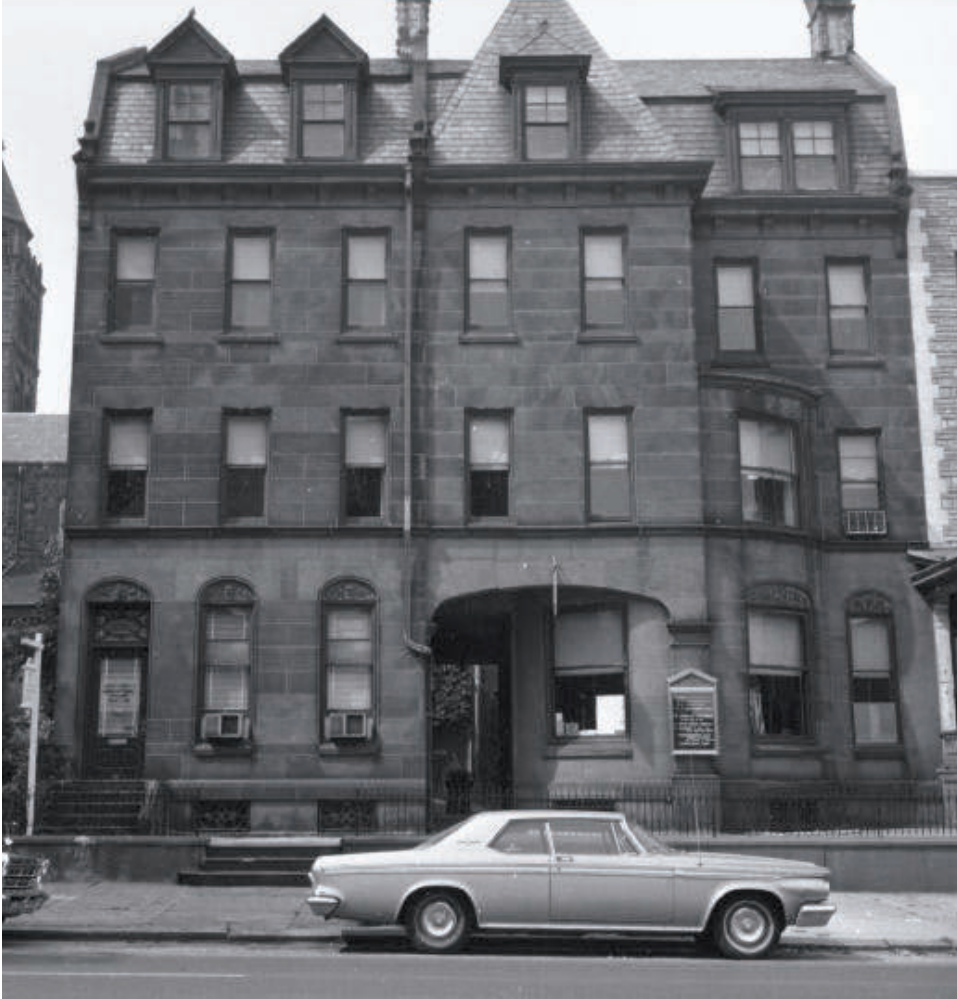
Figure 17 | Elevation of the Parish House. Source: City of Philadelphia Department of Records, Historical Commission Collection, 1969.
