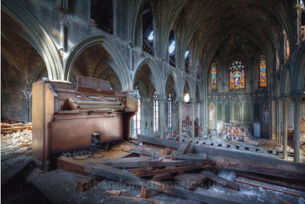
Figure 11 | Interior conditions today require substantial investment to repair the structure for reuse. Source: Michael Christopher, Abandoned America , 2012.
