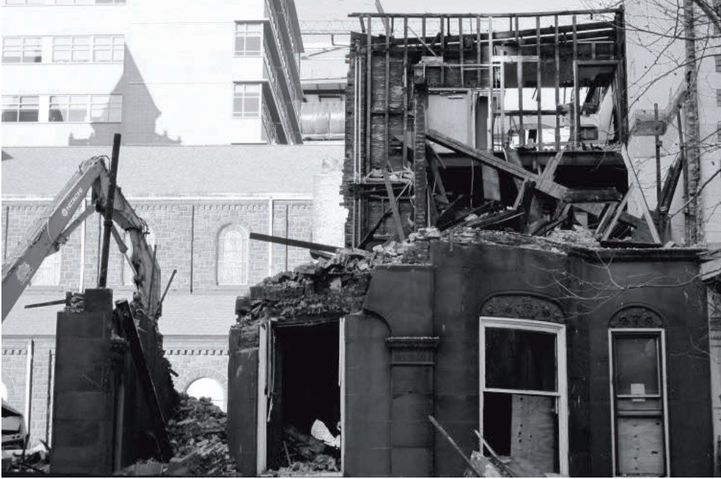
Figure 19 | Parish House demolition. Source: PlanPhilly , 2012.
