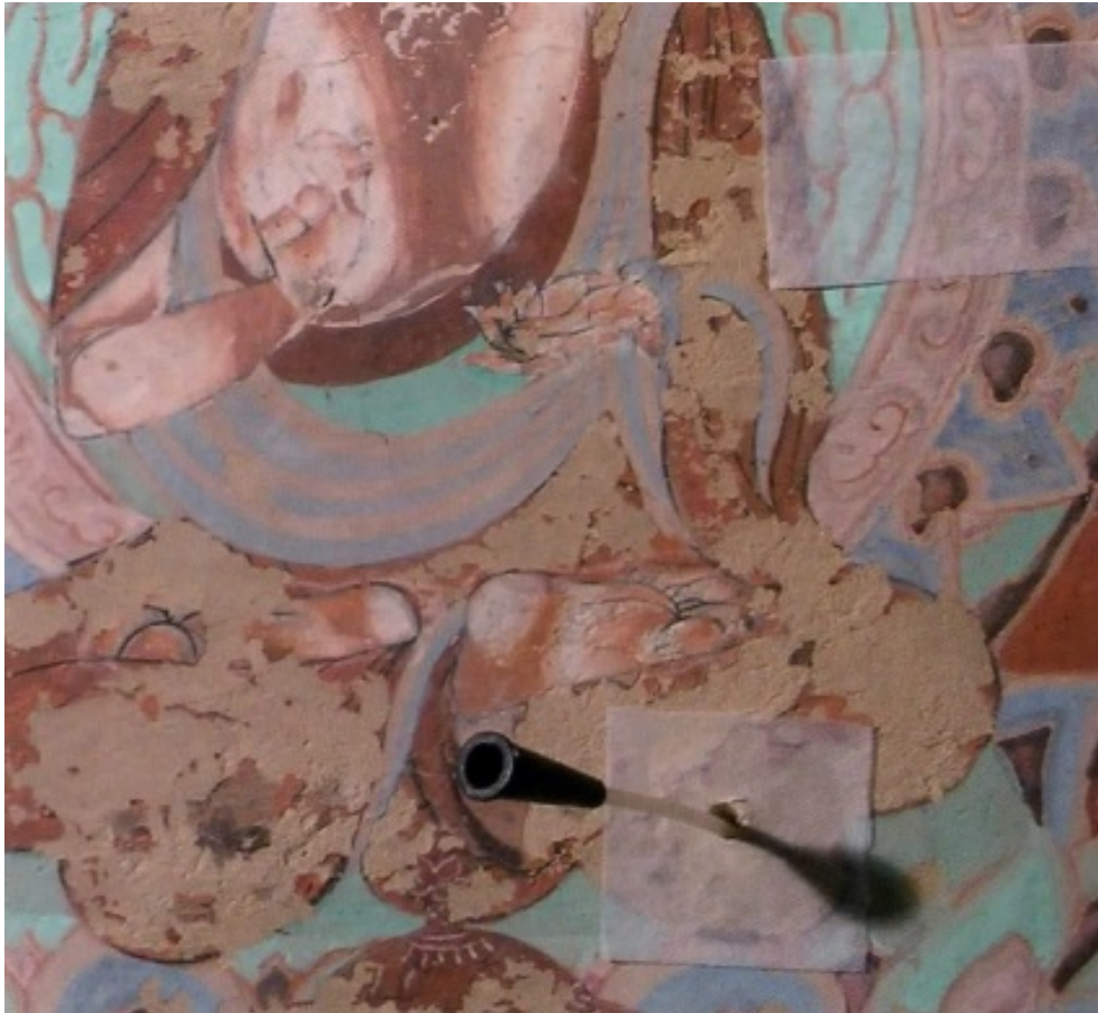
Figure 53. Mural painting in cave 85 of the Mogao grottoes stabilized with temporary facing prior to grouting. Source: Stephen Rickerby et al. Los Angeles: The Getty Conservation Institute, 2010.
