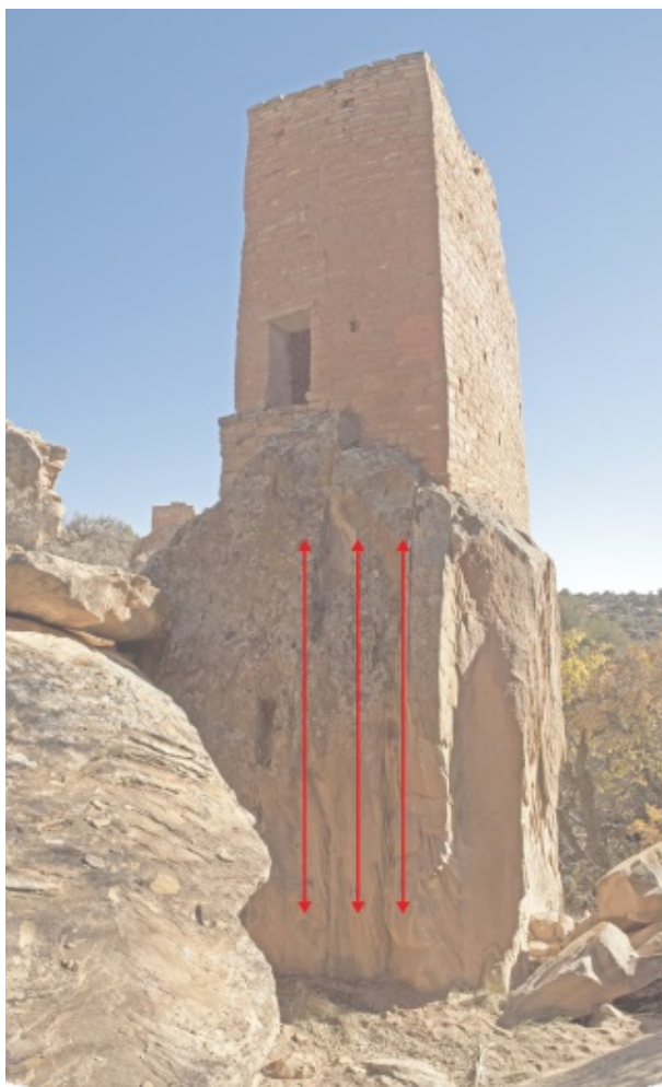
Figure 5. Vertical bedding orientation of the Holly Tower support rock. Source: Architectural Conservation Laboratory, University of Pennsylvania, 2012.
