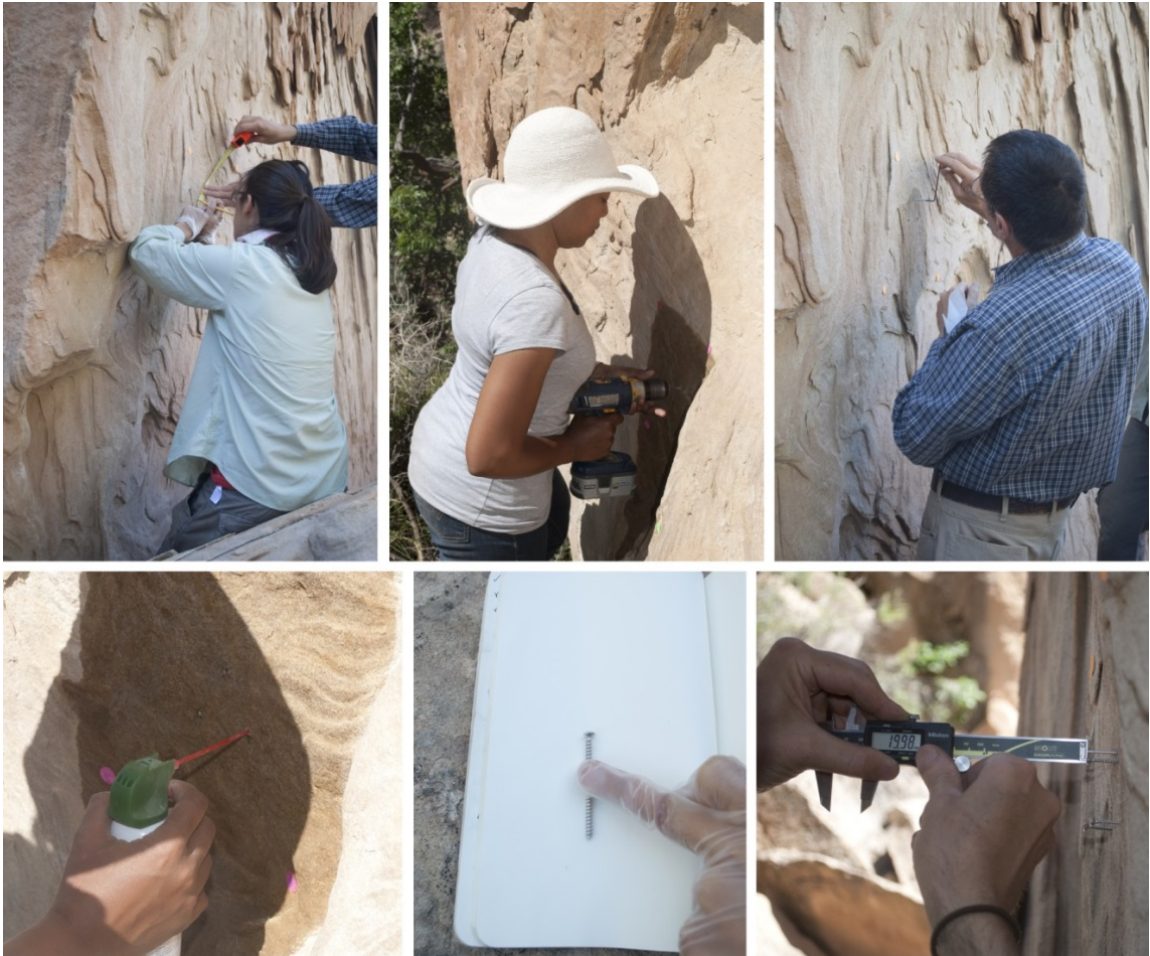
Figure 12. Installation of stainless steel pins to monitor surface erosion. Sources: Laura Lacombe, Milot Berisha and author, 2013.
