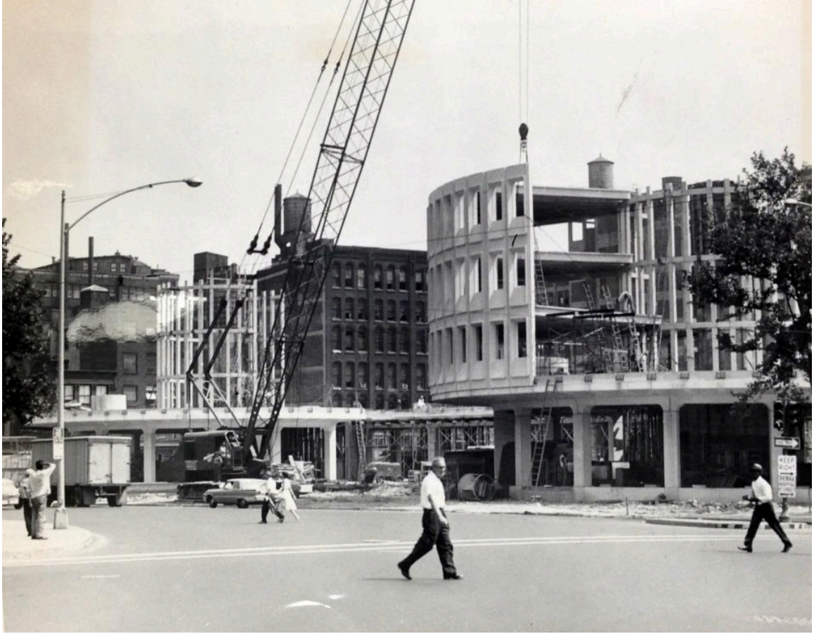
Figure 24. Philadelphia Police Administration Building under construction. 1962. Temple Urban Archives.
