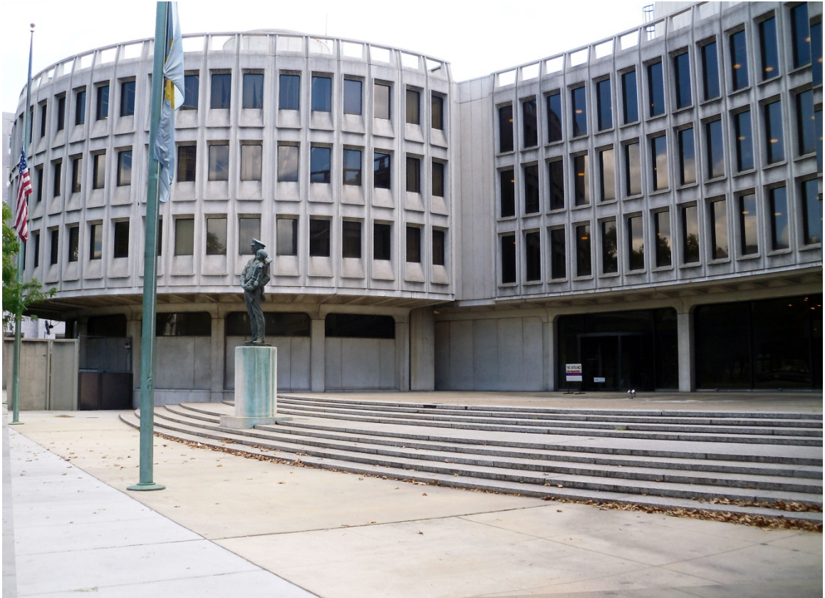
Figure. 30. Shortly after the police began operations in their new building, the main entrance was closed and the entrance moved to the south side. As a result, the plaza sits vacant and unused. The plaza was praised by Architect Robert Geddes for serving as both the functional and symbolic center of a community. Allee Berger. 2012.
