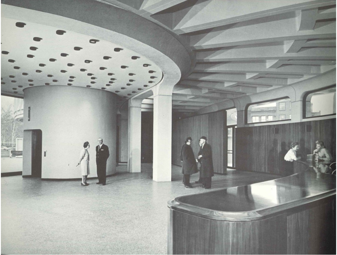
Figure 29. This image of the lobby highlights its open floor plan and attention to curved forms. Earle D. Oakes Collection, The Architectural Archives, University of Pennsylvania
