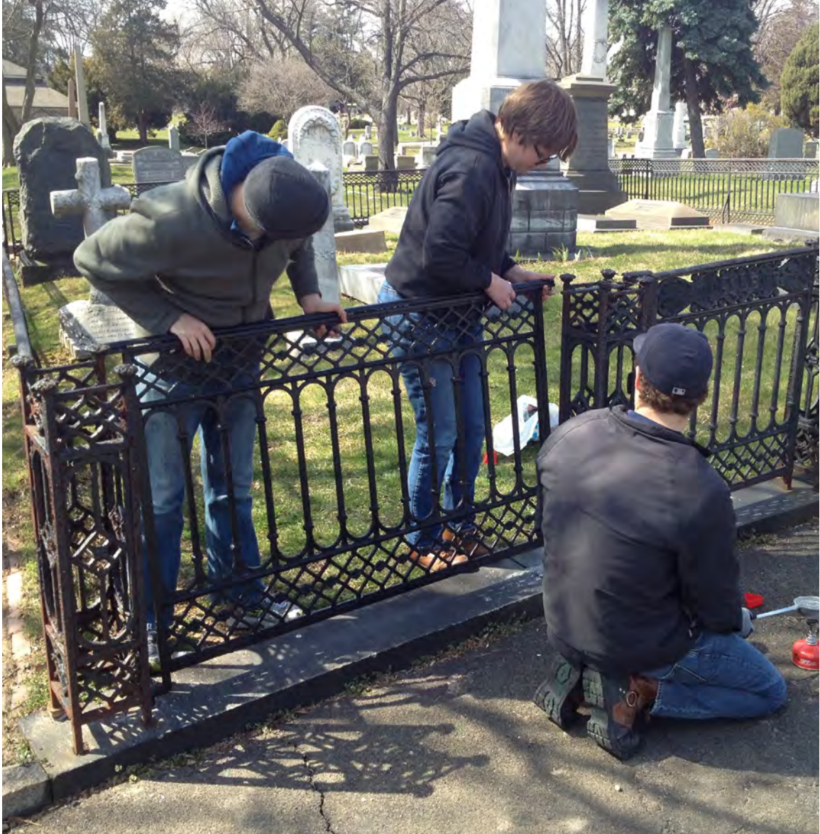
Figure 2.12. Dallett lot restored fence reinstallation.
