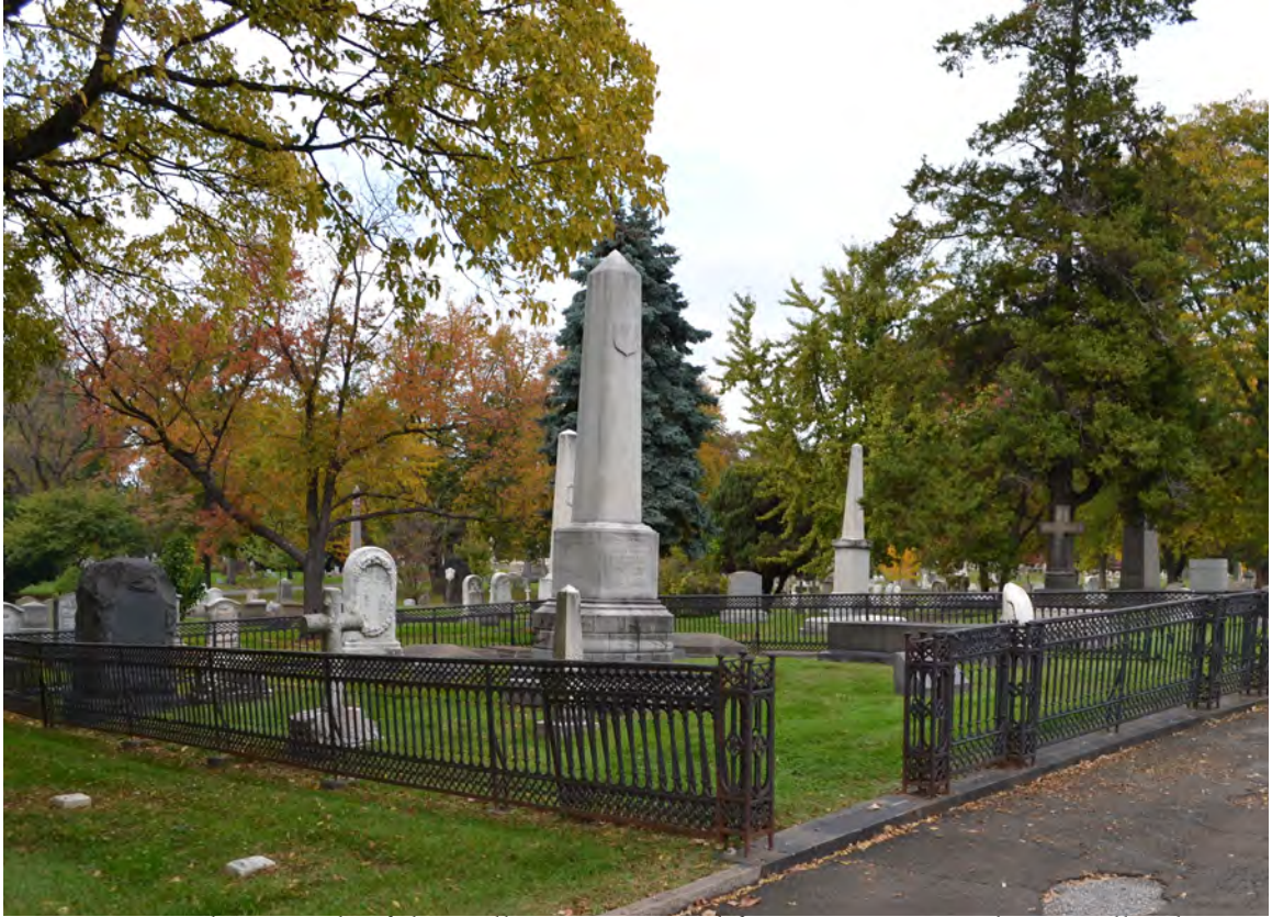
Figure 2.1. A photograph of the Dallett Lot targeted for restoration at The Woodlands. Note the deteriorated condition of the enclosure, including the dislodged section at front. The historic planting scheme has been replaced by a simple lawn, and the access routes have become covered in sod.
