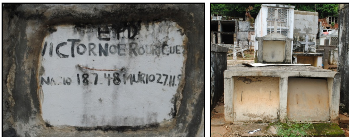
Figure 6-10. The front of the tomb on the left demonstrates how the cement slabs are sealed onto the tomb. Both show a rebar "handle" protruding from the front (SCS CAT 441 on the left and 401 on the right; photograph by author).
