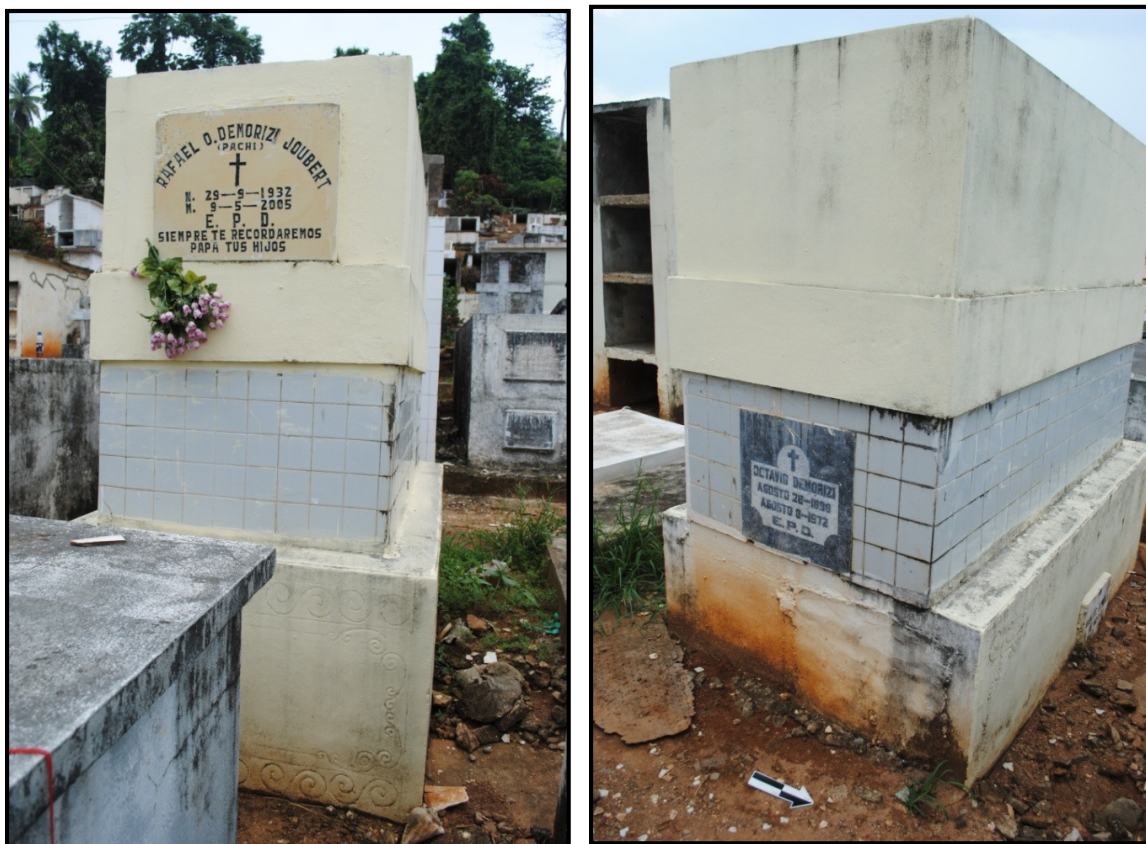
Figure 6-14. The bottom level of SCS CAT 835 displays the swirl motif of the first phase of the cemetery as well as evidence of the back wall being altered to allow for new interments. Based on materials and construction techniques, two additional levels were added to the original tomb well after the earliest phase of use of the Samaná Cemetery (photographs by author).
