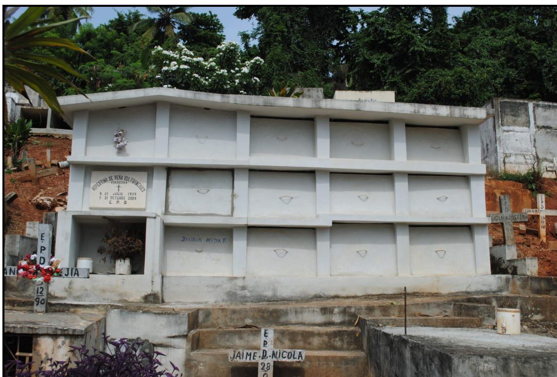
Figure 6-16. The vaults on the right side of this tomb have slabs sealing them, yet there is visible space above the slabs. At least four vaults on the left side of the photograph are fully sealed and marked with the names of the deceased (SCS CAT 1258; photograph by author).
