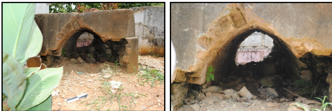
Figure 6-6. View of the vaulted interior and brick and mortar construction of the older tombs in the Samaná Cemetery (SCS CAT 1466; photographs by author).
