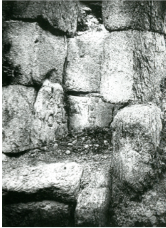
Figure 3.3. Archival photograph of De Rosa's excavation on the Clivus Palatinus. The inscription is visible on the lower facing blocks of the channel. Cecamore 2002 fig. 26.
