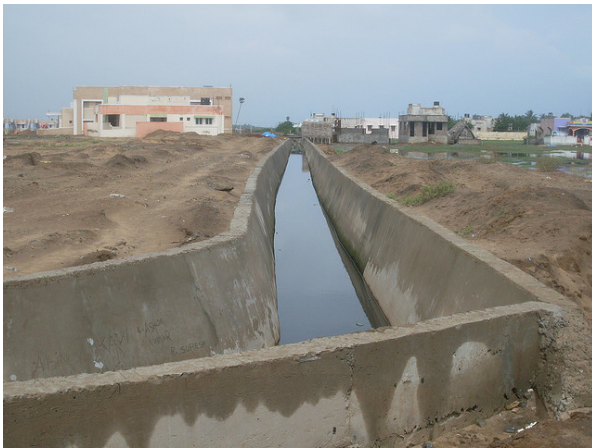
Illus. 5.7 MP Nagar U-drain, looking north
