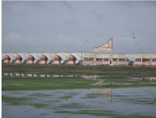
Illus. 5.10 MP Nagar, southern approach
