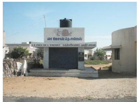
Illus. 5.13 Water filtration facility
