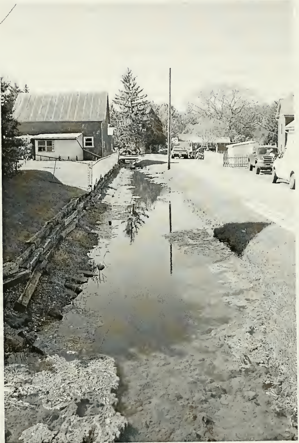
Figure 5: The millrace for Philip Scholl and Daniel Grim's gristmill looking south away from the mill.
