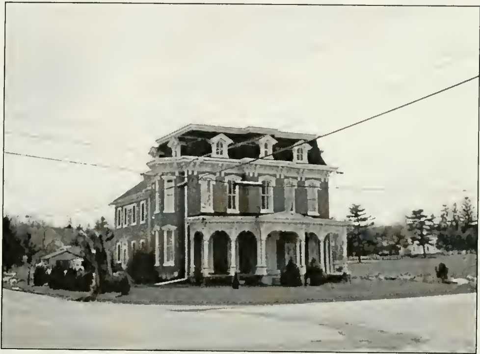
Figure 36: View of the Edwin DeLong house looking south. The Second Empire portion of the home was added to George Seibert's stone farmhouse visible behind the brick portion.
