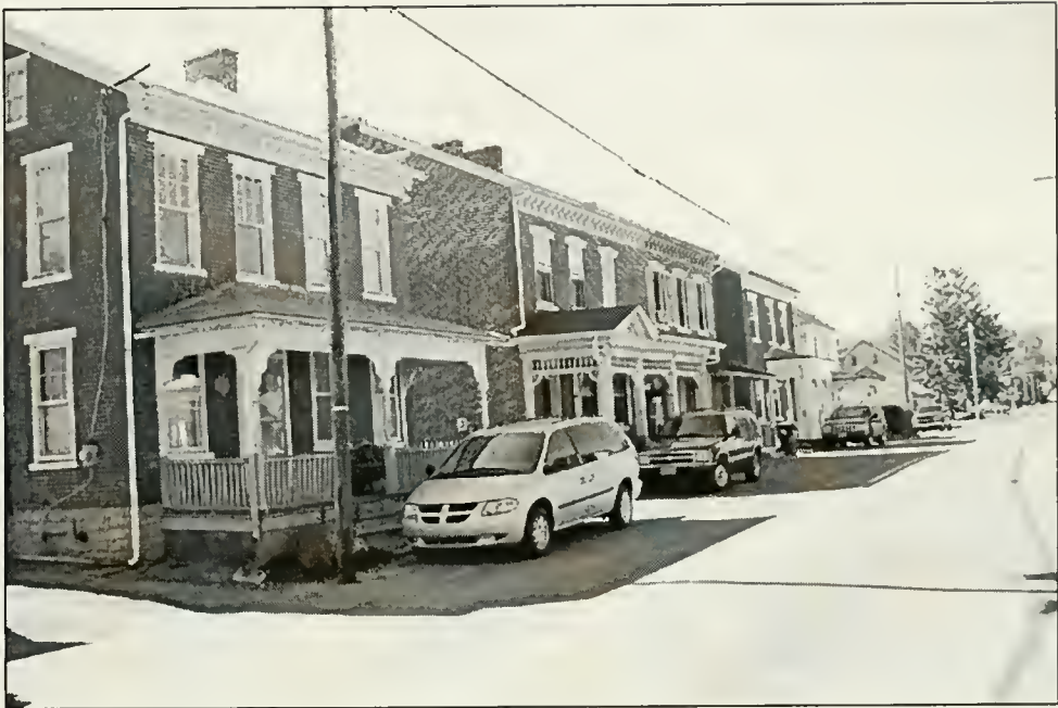
Figure 53: Looking south along Bowers Road.
