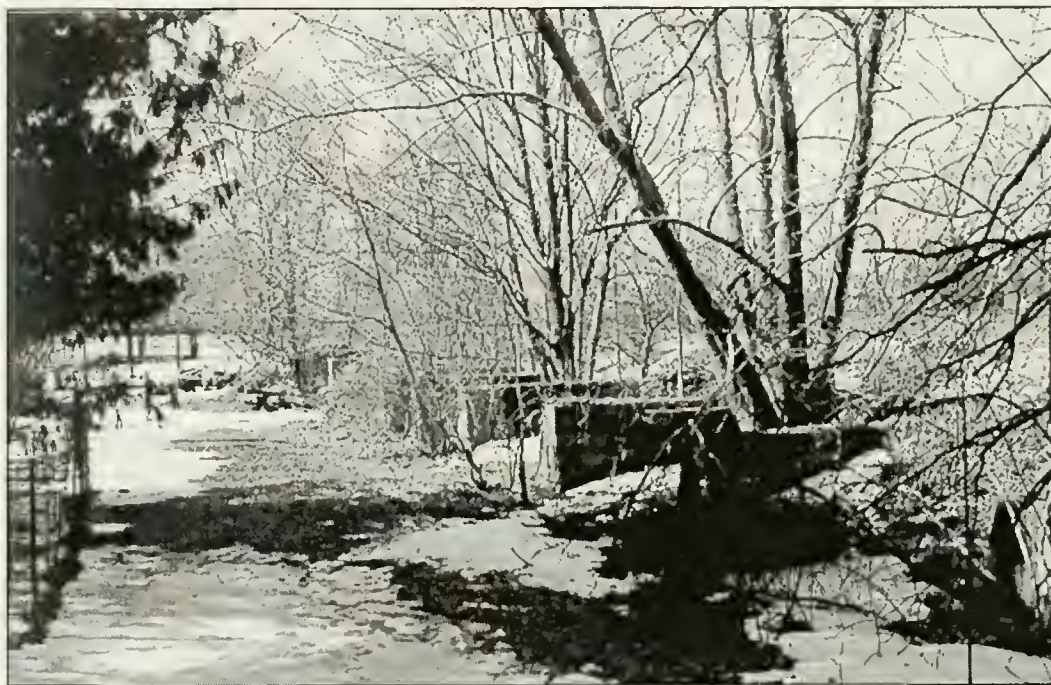
Figure 42: These concrete piers once supported a railroad siding used to import and export goods in Bowers.
