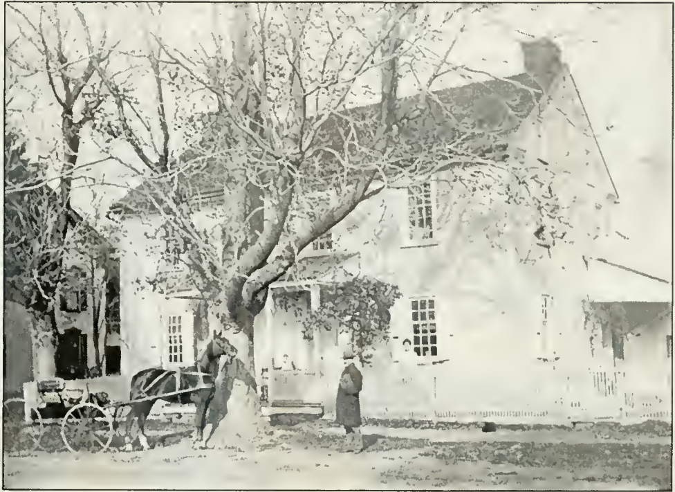
Figure 25: The parsonage and schoolhouse adjacent to the church, 1905. Pennsylvania State Archives, Arthur Bransky Collection.
