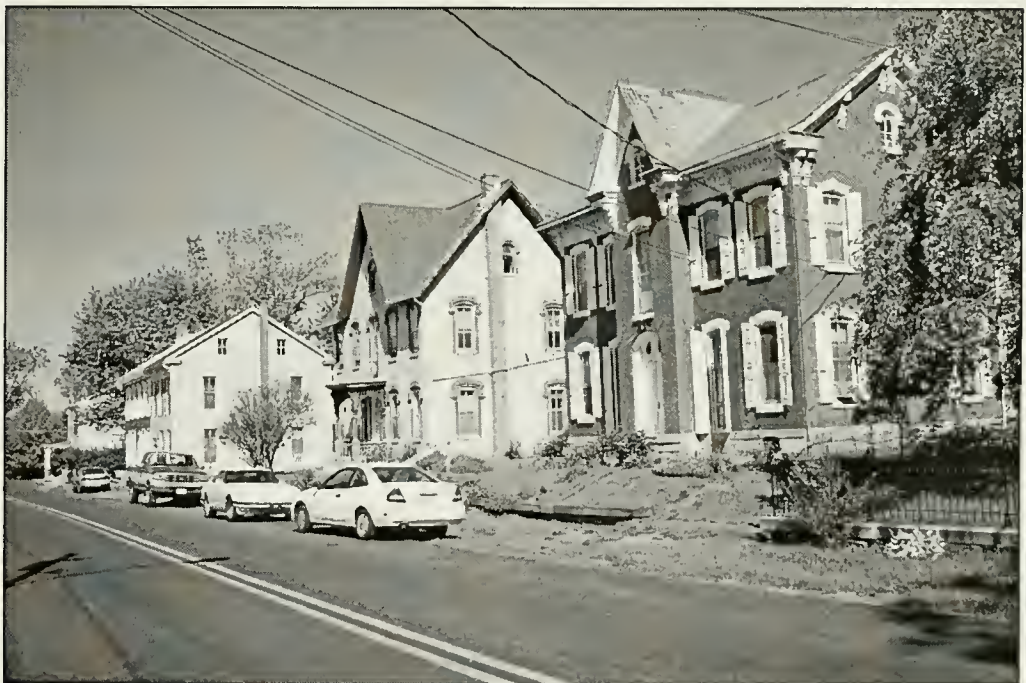
Figure 12: Looking west along Old Bowers Road. At right are two of the large mansions built by wealthy farmers and merchants around 1875.
