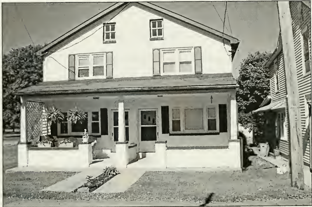
Figure 27: The 1874 schoolhouse as it appears today.
