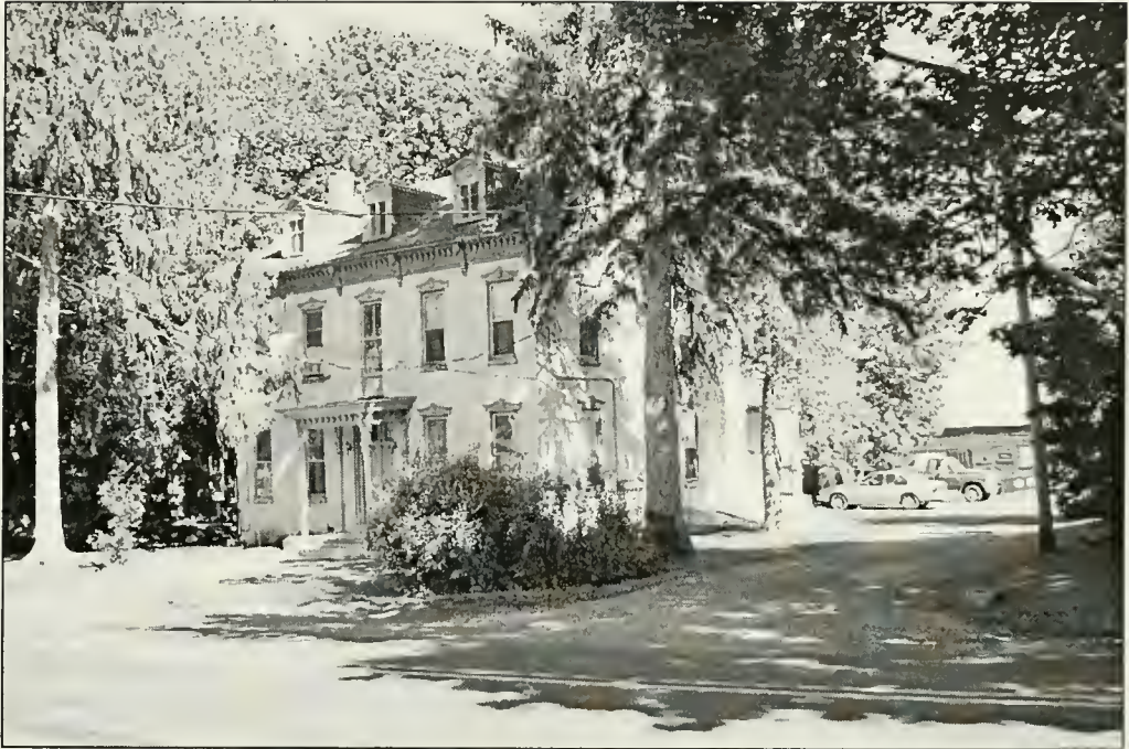
Figure 11: William Sharadin constructed this large mansion around 1870 on land once farmed by Daniel Grim.
