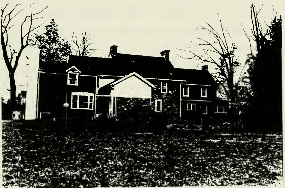
Figure 7. Haldeman House. North elevation [photo by author].
