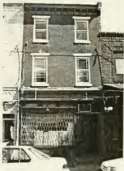
Figure 2-M: Insertion of Display Window
