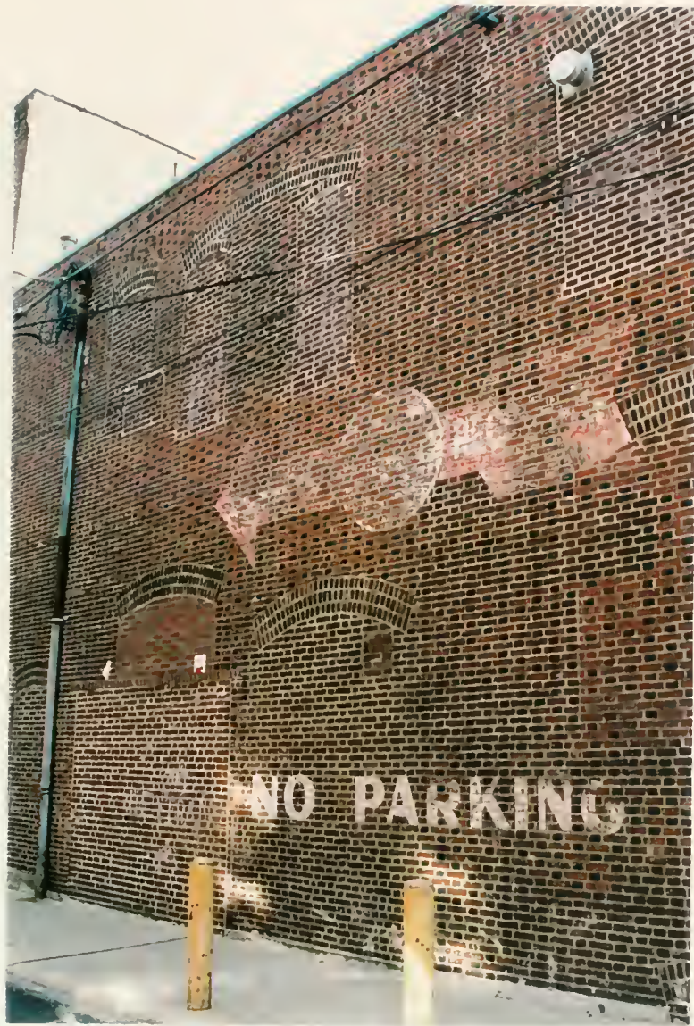
Figure A-11: Detail of Side Wall at 1025-1021 S. Ninth Street
