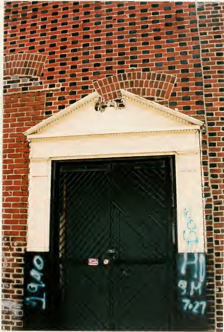
Figure A-14 Details of the side wall of 1025 - 1021 S Ninth Street
