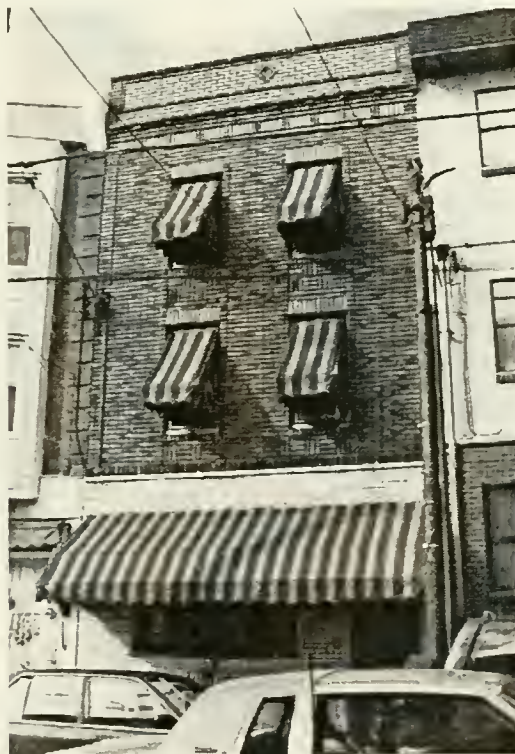
Figure 2-C: Example of façade with multiple materials - 742 S. Ninth Street
