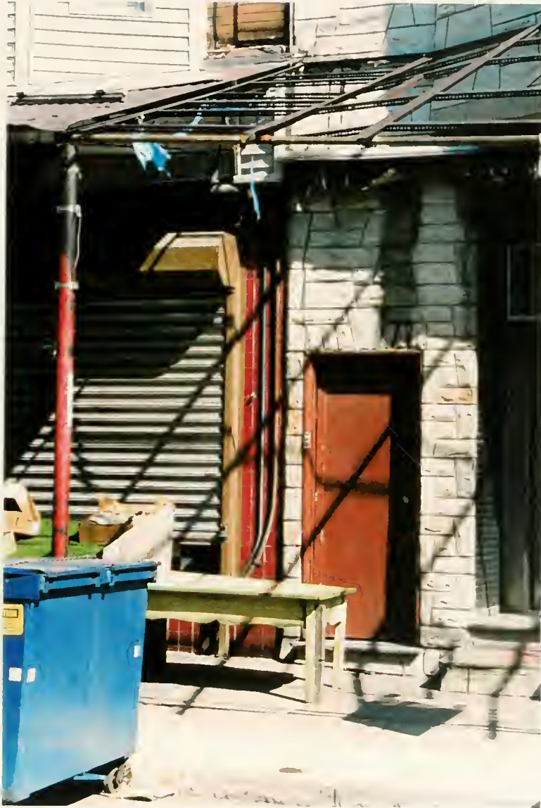
Figure A-16 Detail of Facade Materials along Ninth Street
