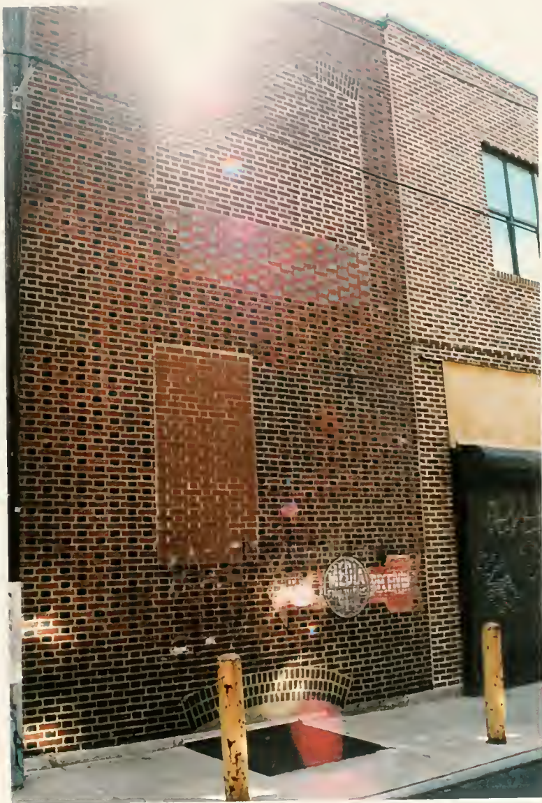
A-12: Details of side wall of 1025 - 1021 S. Ninth Street
