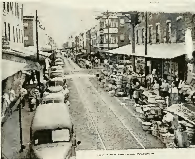
Figure 3-B: 1952 view of Ninth Street. Note the vendor trash taking up a lane of traffic (Courtesy of Temple University, Urban Archives, Philadelphia, PA)
