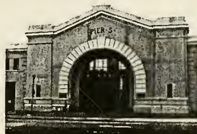
Fig.16. The bulkhead at Pier 5.
