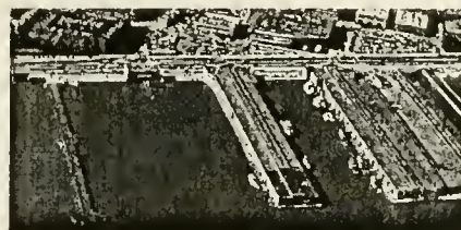
Fig.34. An alternating pattern of finger piers and water
