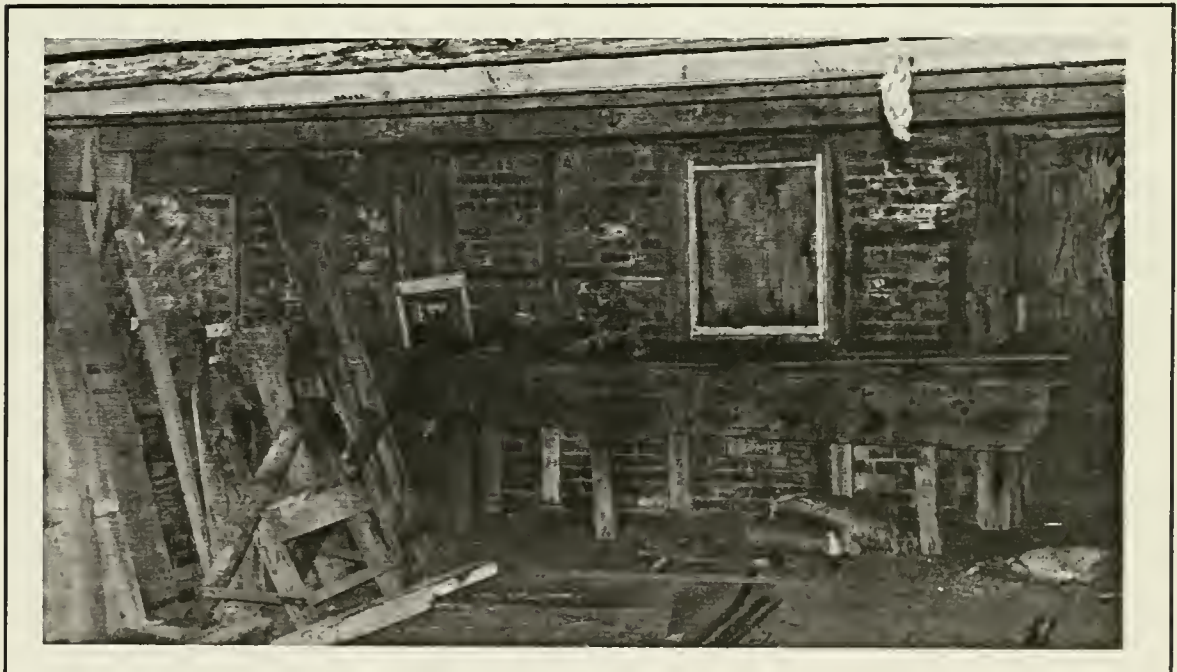
Fig. 29 Horizontal and vertical half-timbering of the east wall.
