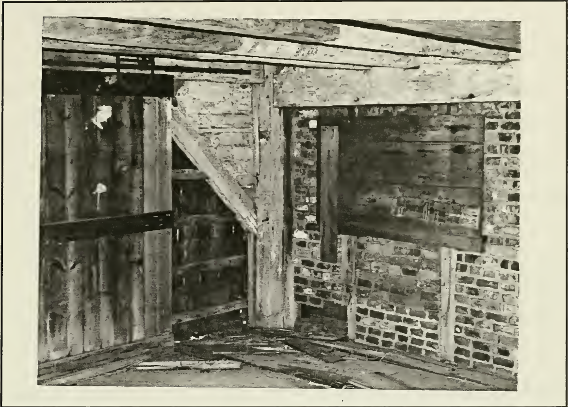
Fig. 30 Evidence of original sunbaked bricks, see north west corner where the bricks are white washed.
