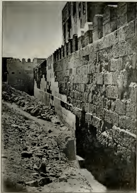
Figure I.7 Tower 4 after Comité reconstruction, 1951.
