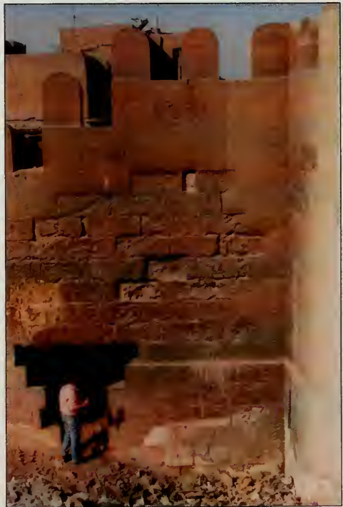
Figure 1.9 Segment of the city wall showing construction technique, running and Flemish bonds.
