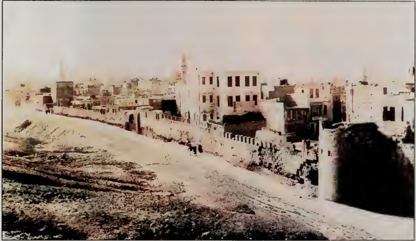
Figure 1.4 View of the eastern portion of the Ayyubid city wall of Cairo from the Darassa hills with the former Darb Shoughlan School noticeable in the center of the photo. Note the extensive loss of veneer stone in certain areas of the wall.
