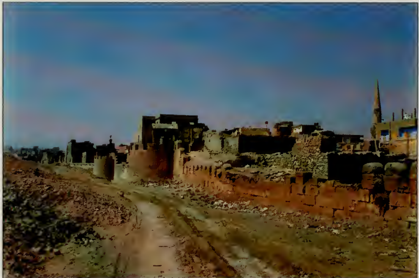
Figure 1.5 Similar view of city wall of Cairo in 1998 with the former Darb Shoughlan School in the center of the photo. Note the higher grade level, the reconstruction of one tower and crenellation by the Comité.
