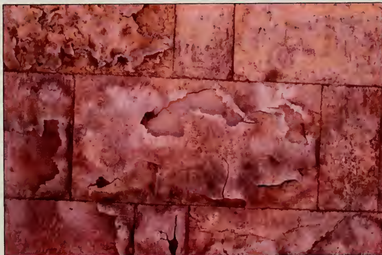
Figure IV.10 Detail of the thin salt crusts (veil) falling off in large plaques from the surface of the stones, 2000.
