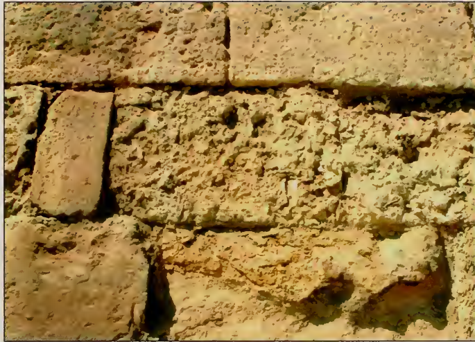
Figure 1.11 Differential weathering of the veneer stones of the city wall.
